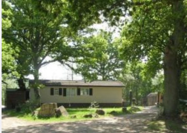
Unlawful encroachments at Shortheath Common, Hampshire
