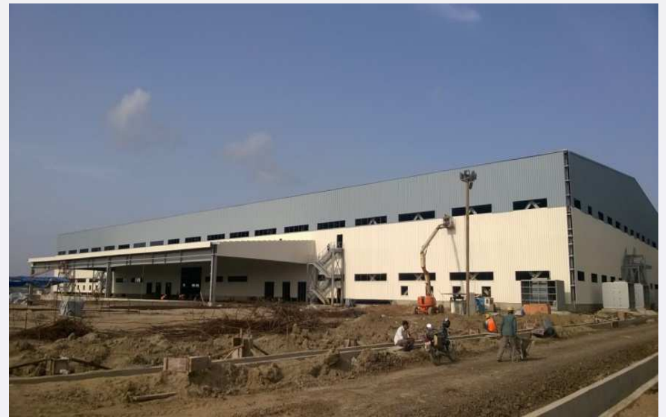
Pic 4: Warehouse Building
