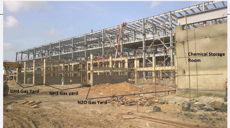
Pic 2: Main Manufacturing Building
