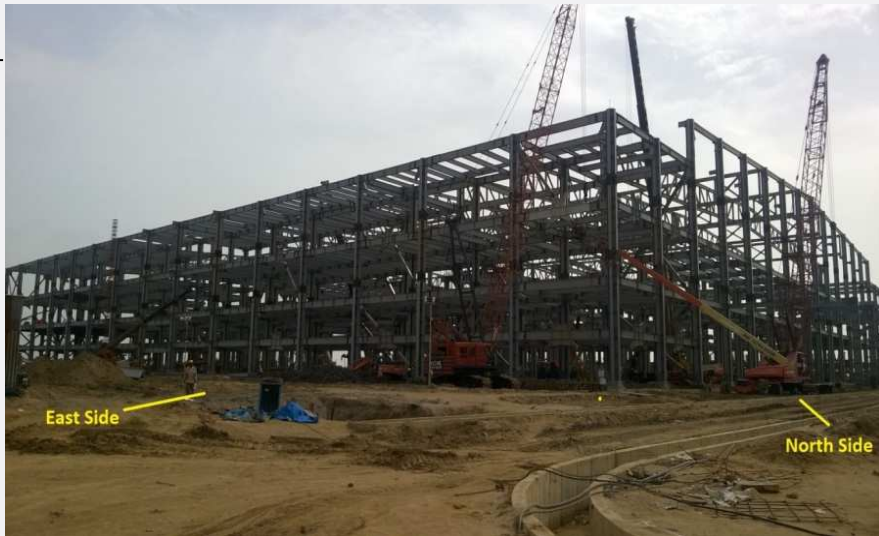
Pic 1: Main Manufacturing Building
