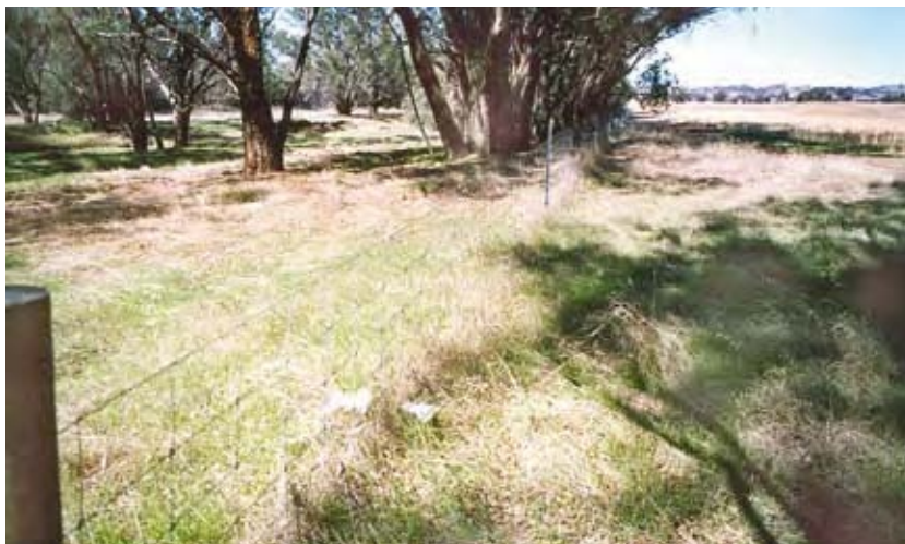
Fence condition: GOOD.
