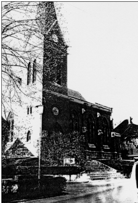
Fig. 36: In August 1976, the Protestant church at D-96484 Meeder-Wiesefeld was fumigated with Zyklon B. Subsequently, blue-colored stains appeared all over the plaster (see Fig. 37).
