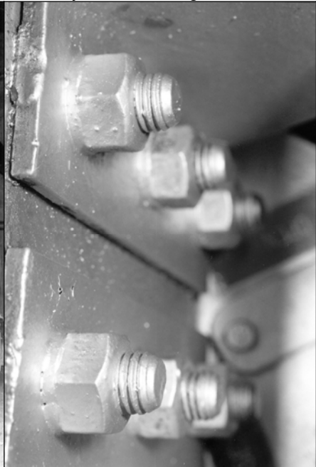
Fig. 95: Closeup of bolts on door hinges.
