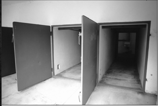
Fig. 26: Doors of professional delousing chambers (DEGESCH circulation chamber) at the Dachau camp.
