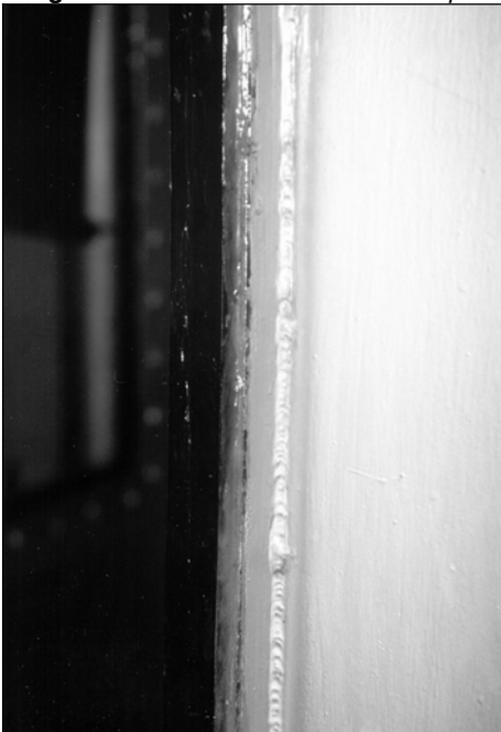
Fig. 90: Closeup of rubber seal around gas chamber door, also covered in vaseline when in use.
