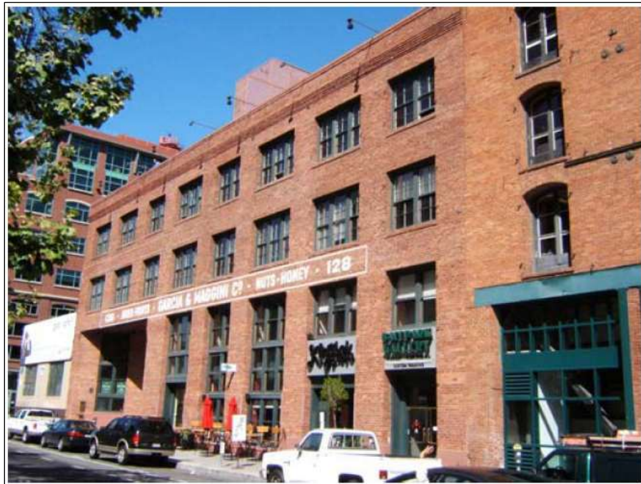
Garcia and Maggini Warehouse, 128 King Street
