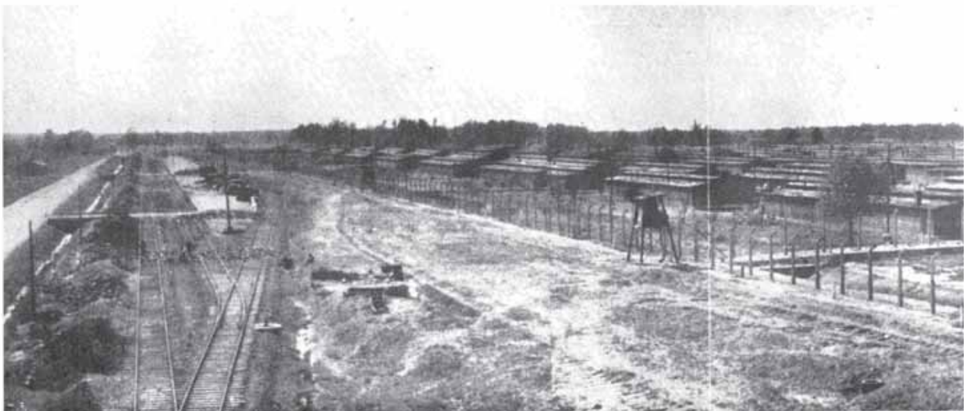
Photo 2 – Taken by Soviets, 1945: (below) From on top of the entrance gate looking west along the unloading ramp.
