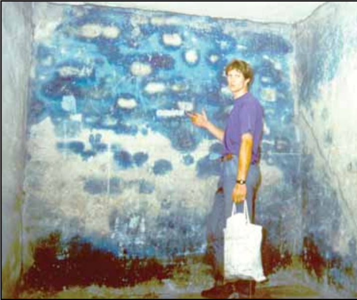
Photo 1: Interior wall of the disinfestation wing of Building 5a at Auschwitz-Birkenau
