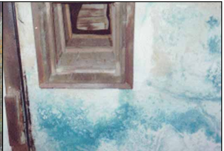
Photo 4: Ceiling of the make-shift disinfestation chamber in "Bad & Desinfektion I" at Majdanek.
