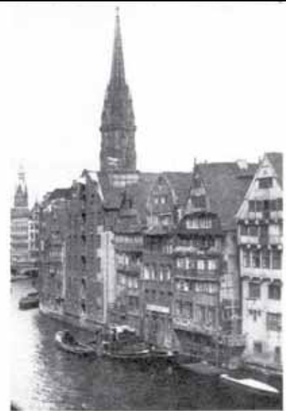
Photo 2: The Nikolaifleet waterway in the Altstadt before the 1943 bombing.
