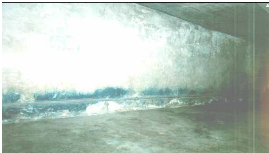
Photograph XIII: Disinfestation facility, Barrack 41, Chamber III, east wall.
