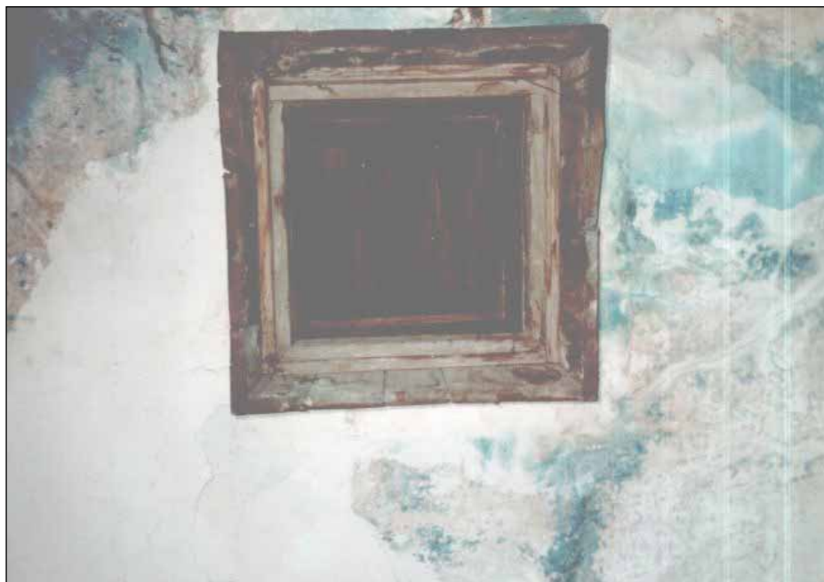
Photograph XVIII: Barrack 41, gas chamber, western opening in the ceiling. © Carlo Mattogno
