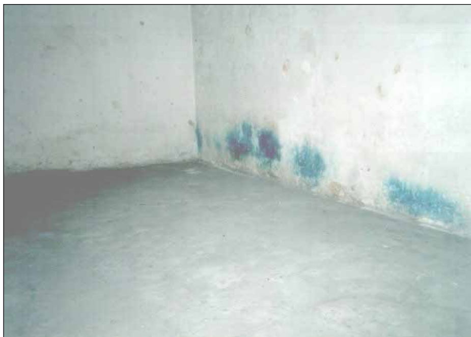
Photograph XIV: Disinfestation facility, Barrack 41, Chamber II, west wall.
