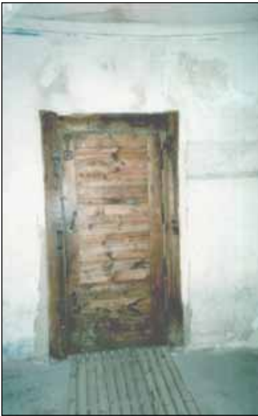
Photograph XVI, XVIa: Barrack 41, gas chamber, south door. In the left part of the door there are three latches which are inserted into the three corresponding hooks on the door frame via handles operated from the other side of the door (Photograph XVIa). © Carlo Mattogno
