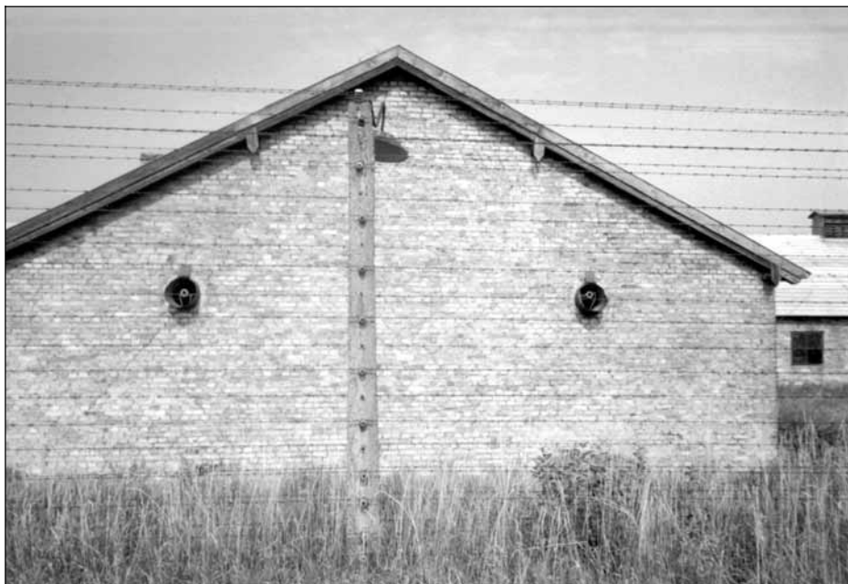
1. Birkenau, BW 5b, round openings for placement of ventilators in the outside wall of the gas disinfestation chamber. July 1992, © Carlo Mattogno.
