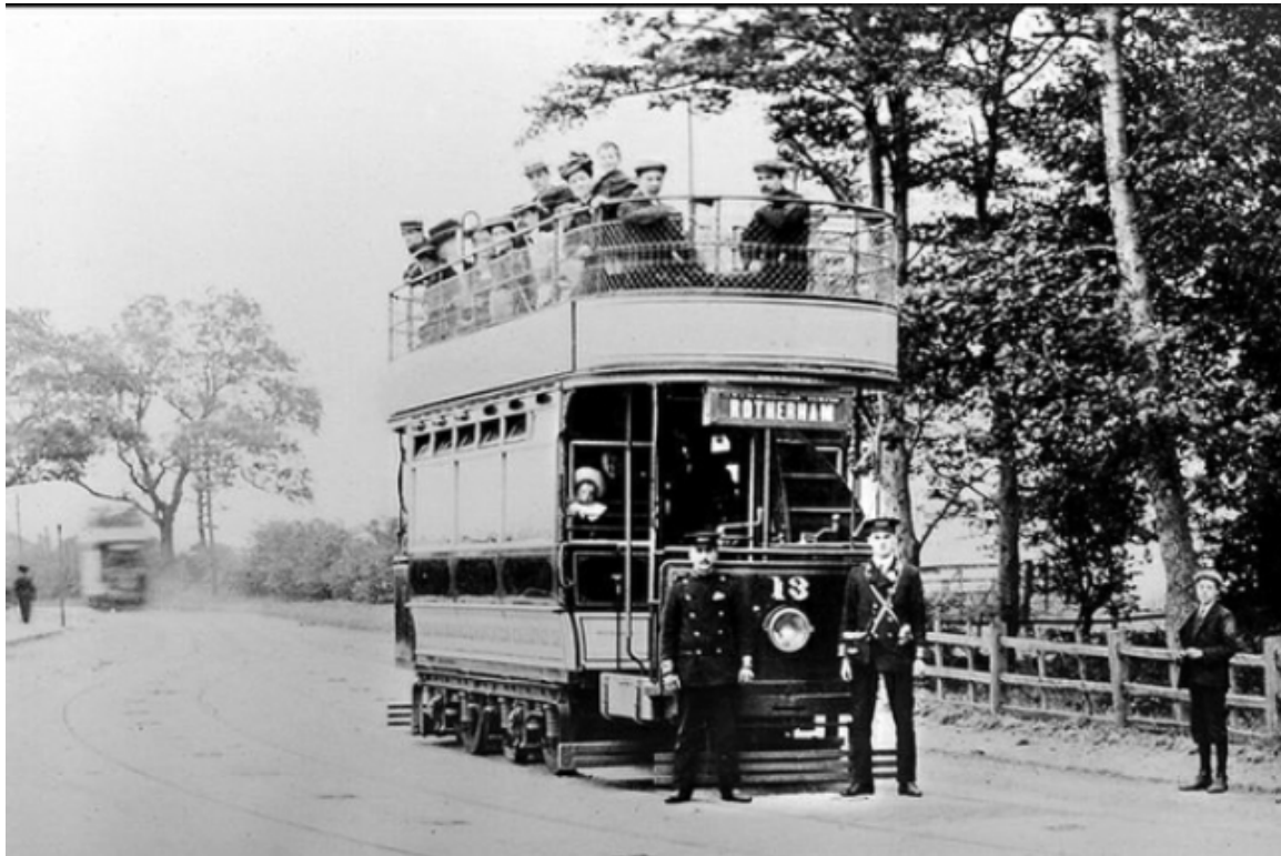
No. 13 was a double-deck open-top 4-wheel car on Mountain & Gibson trucks dating from 1907. It was fitted with a top cover in 1908 and withdrawn by 1929. (LTHL collection).
