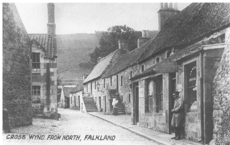
Cross Wynd in the early 20 th century, a dense urban area showing many of the characteristic features of the historic Falkland townscape
