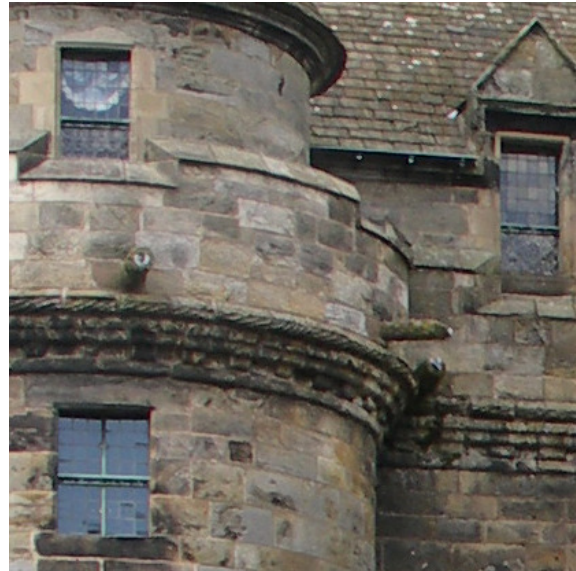
Coloured timber windows are historically appropriate.
