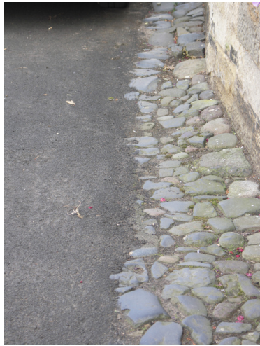
Tarmacadam lacks the scale and local character of the cobbles it covers.
