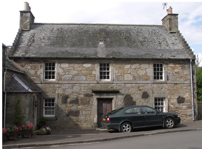
Mixing slate types during repairs should be avoided.
