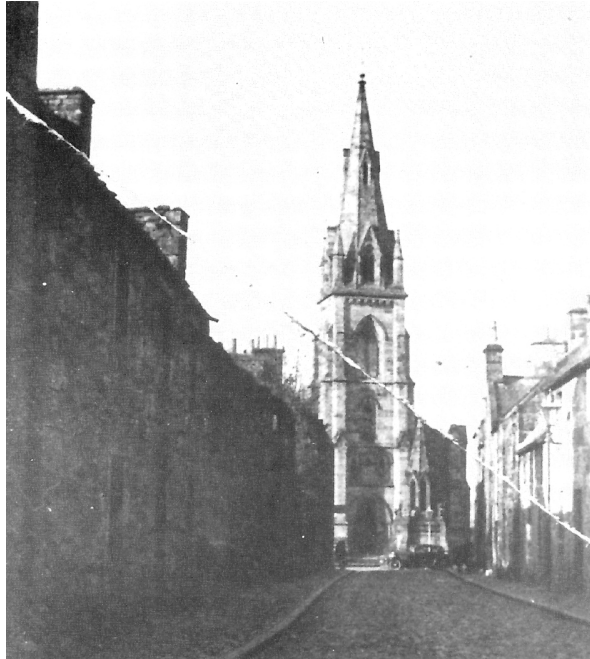
Cross Wynd showing later pavements and street with stone setts and underground drains.
