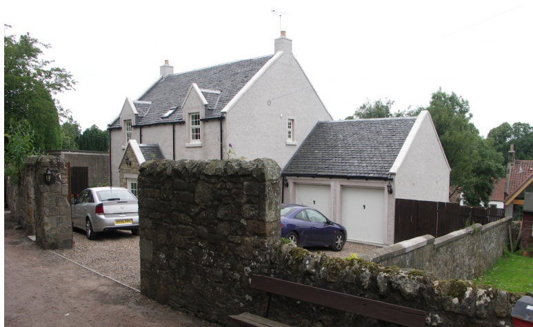
Modern backland development replaces the historic burgh boundary wall and rigg garden with development that is suburban in character.
