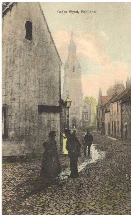
Cross Wynd showing surface drainage over cobbles.
