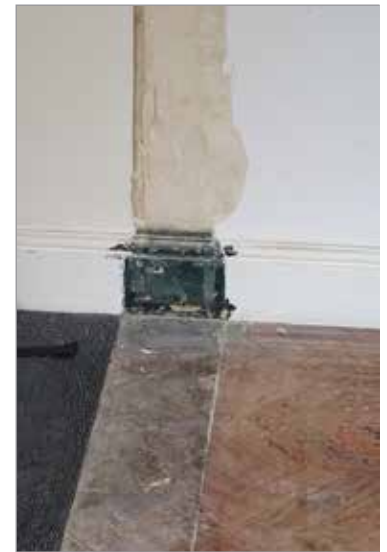
4. Removal of the centre partition wall reveals original paint colours in the Servants' Hall
