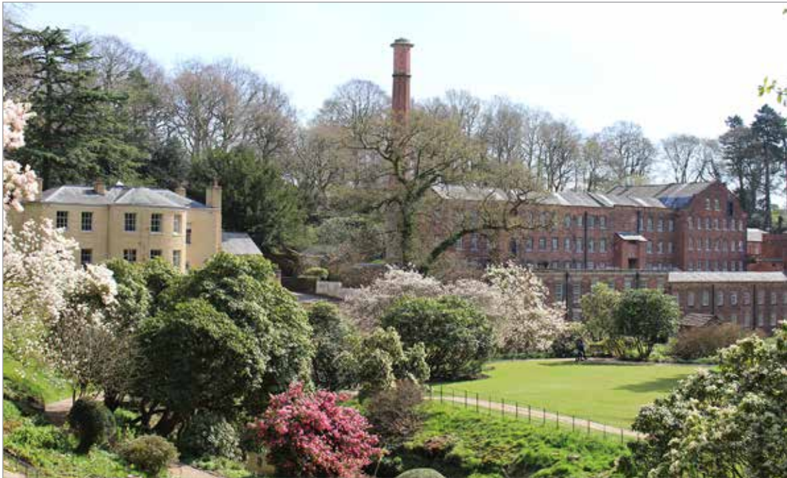
3. The mill and Quarry Bank House
