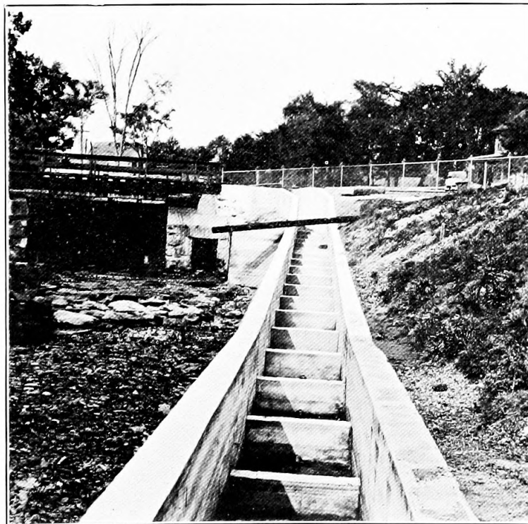
FIG. 12. — Standard straight-run fishway of concrete, Stanley Iron Works, Bridgewater.
