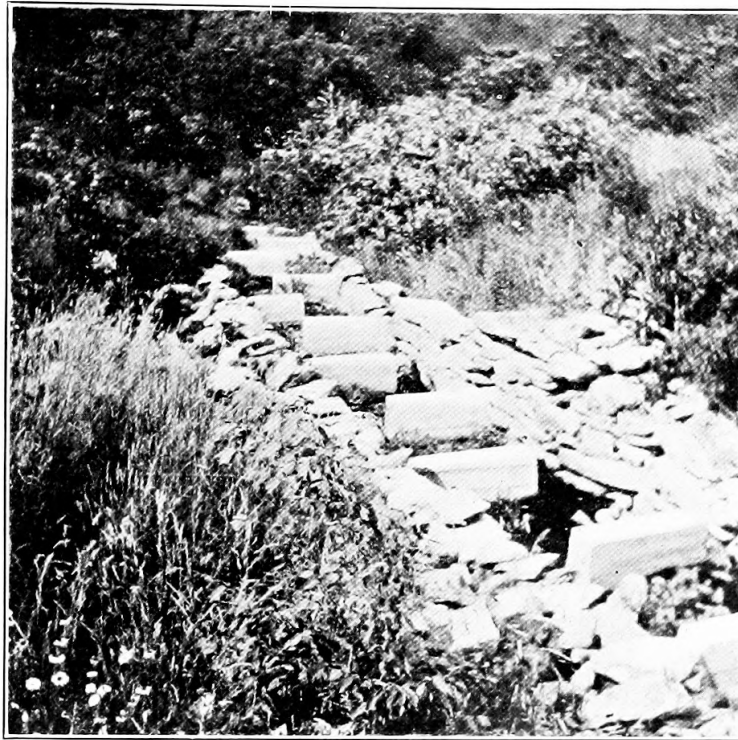
FIG. 11. — Stone fishway with concrete baffles, Nemasket River.
