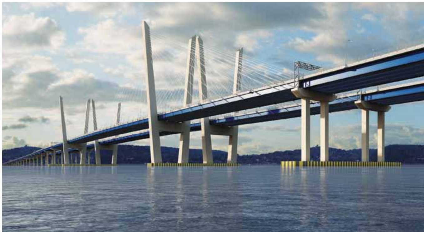
COURTESY OF NEW YORK STATE THRUWAY AUTHORITY
