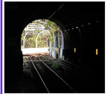
Tunnel Portal at Kings Cross
