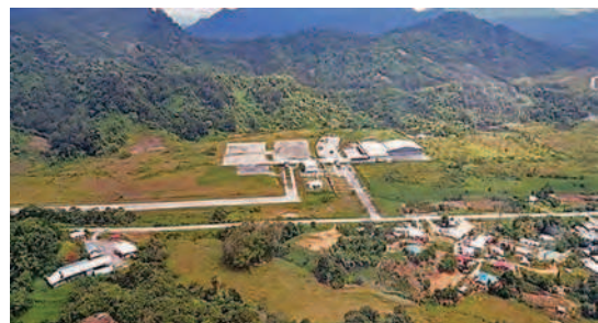
Figure 8.5. Aerial View of Tebedu Inland Port
