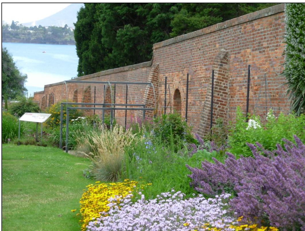
Figure 9.3: Section of western side of Eardley-Wilmot wall 2010.
