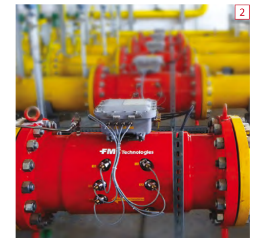
fot. 1. SRP Meszcze, zgodny z MID gazomierz ultradźwiękowy MPU, prod. Integrotech. / Pressure Reduction and Metering Station Meszcze, MPU ultrasonic gas meter, compliant to MID Produced by Integrotech.
