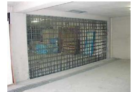
Strengthen building structure by external reinforcing method and buildup of inner wall (conceptual image)
