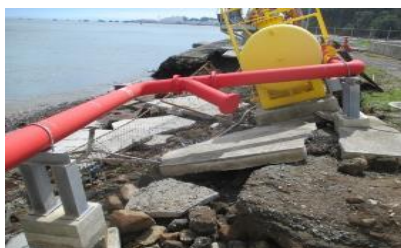
Recovery of damaged SDF facilities
