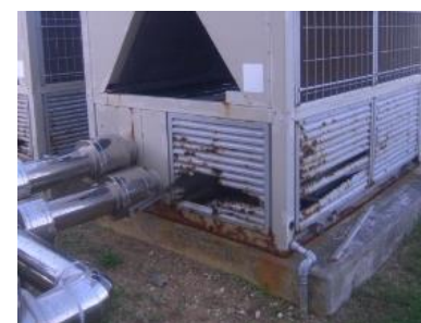
Upgrade Air-Conditioning facility
