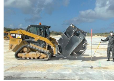
Equipment to Restore Damage in Runways
