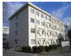
Strengthen building structure by external reinforcing method and buildup of inner wall (conceptual image)
