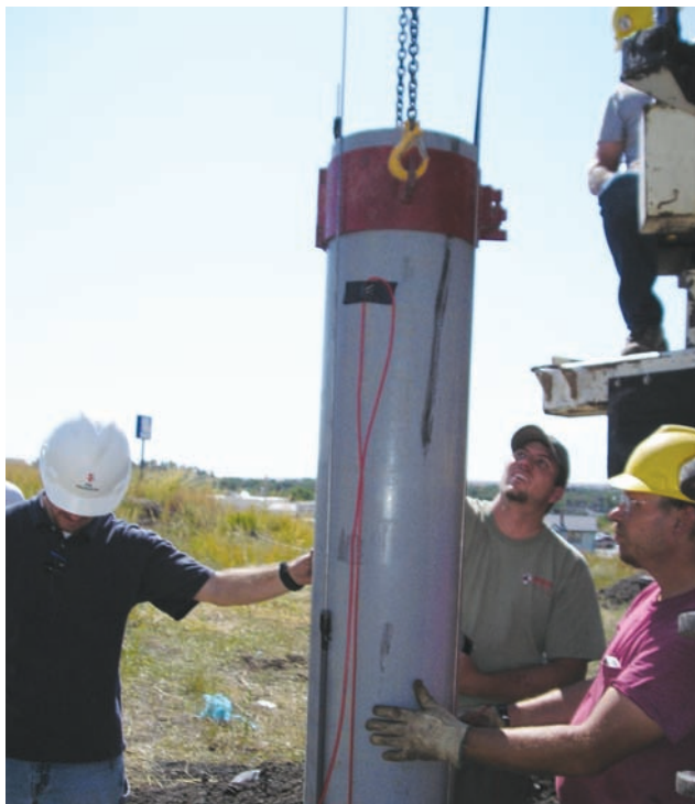
[FIG. 4] Pile being lowered into the shaft.
