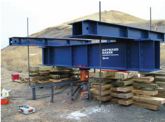
[FIG. 5] Reaction frame setup for static load testing of plastic piles.
