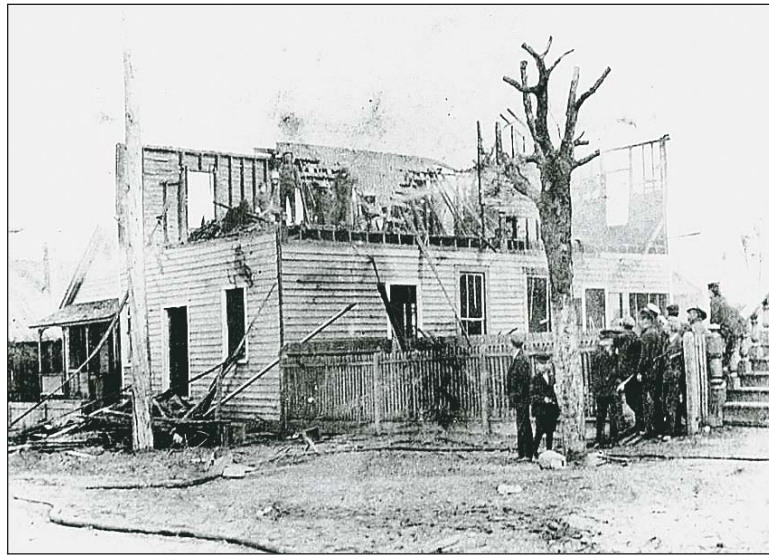
Black firefighters stand on the second floor of the destroyed Love and Charity Hall in Wilmington. Children watch on the steps below. The building housed the city's black-owned newspaper.
