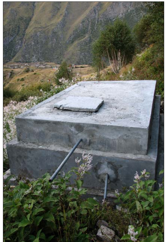
Figure 2.7: Concrete Holding Tank, Second Government Project
