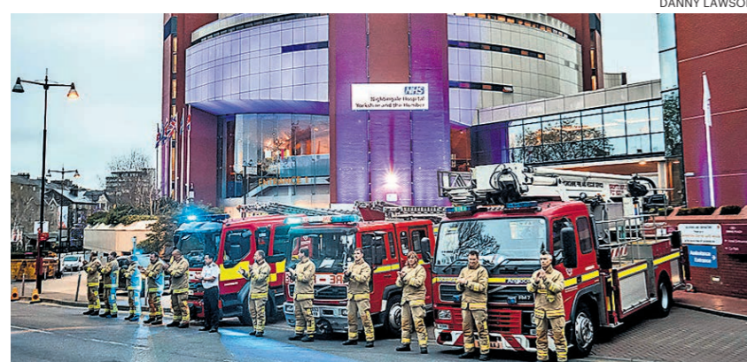
Engineering firm NG Bailey (No 59) helped transform Harrogate Convention Centre into an NHS hospital, installing 19km of pipework and 3,500 sockets
