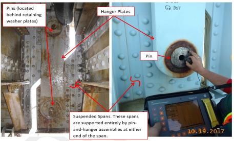
Typical Pin-and-Hanger Assembly (2 Pins + Hanger Plate) Using ultrasonic testing to verify the integrity of the pin
