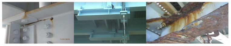
Cracked and Deteriorated Structural Steel. Despite nearly continuous repairs, an aggressive environment affects the steel
