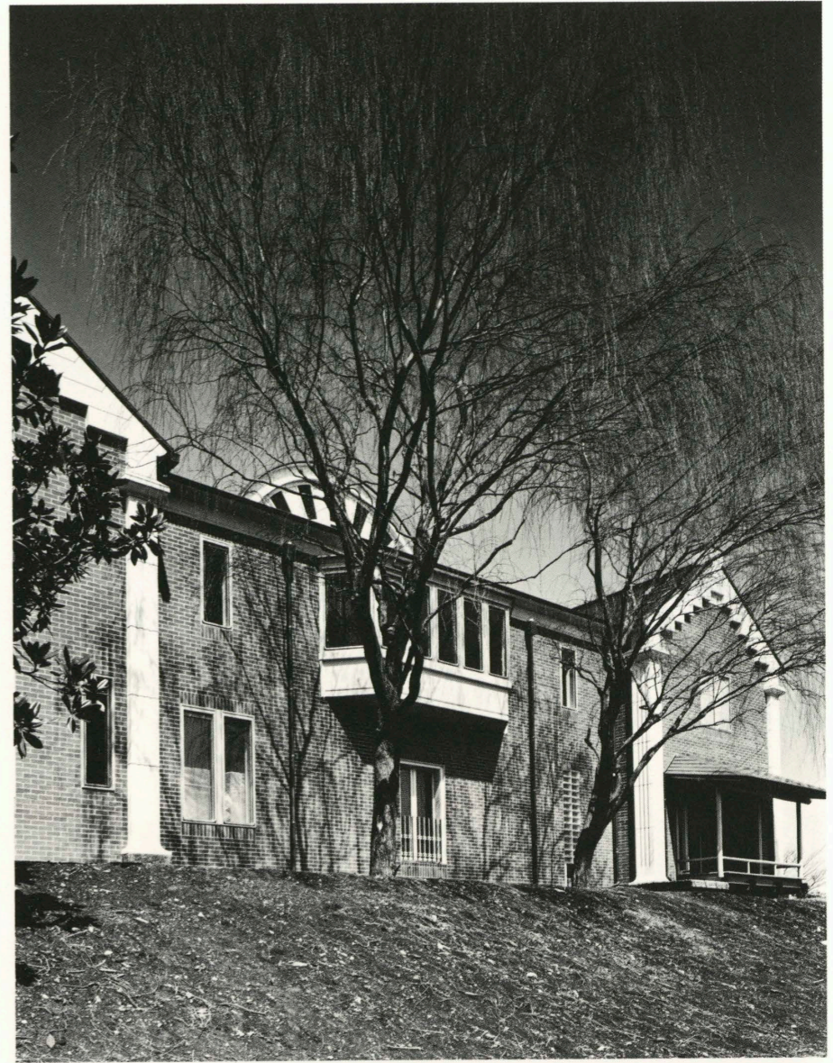
南側外観 Outside view on the south side.
