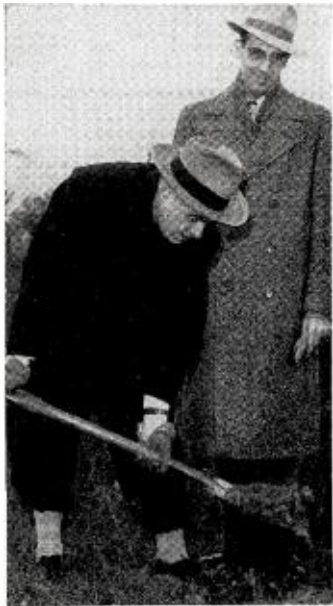
MORE SHOVELING goes on as Capt. Pierre Boucheron, general manager of WGL Fort Wayne, and director of broadcasting division of Farnsworth Television & Radio Corp., breaks ground at the site of the station's new transmitter at Waynedale. By spring station will move from 1450 kc to 1250 kc, on 1000 w. William Aldrich (r), sales manager, seems to be no help at all in the manual labor department.
