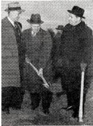
ANOTHER SHOVEL hits the dirt as officials of WFIL Philadelphia signal start of construction of the station's new 5,000 w transmitter in Whitmarsh Township. Roger W. Clipp, WFIL general manager, handles the shovel, while Louis E. Littlejohn (l), chief engineer, and Walter H. Annenberg, publisher of The Philadelphia Inquirer , owner of WFIL, give advice from the sidelines.
