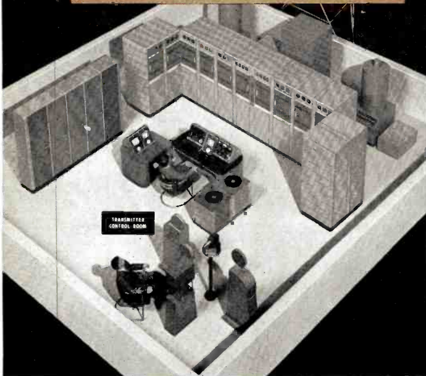
50 kw VHF (ERP range, 50 to 200 kw) Block "U" set-up for RCA's "50-kw." This arrangement is well suited for local building situations—or where physical limitations call for an antenna of medium gain and high ERP. Note film camera control and preview monitor next to operator for his convenience.
