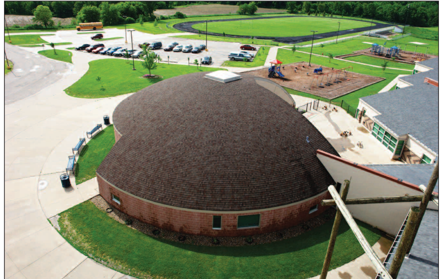
Overhead of the Meskwaki Elementary School
