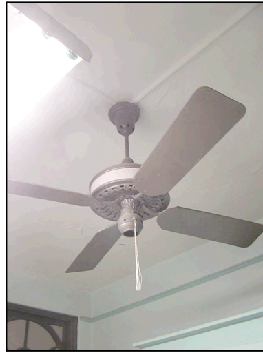
Figure 21: The ceiling fan in the joker stand area appears to be consistent with a ceiling fan identified as part of the 1925 construction of Fire Station No. 9, one of the four sister stations to No. 11. 3
