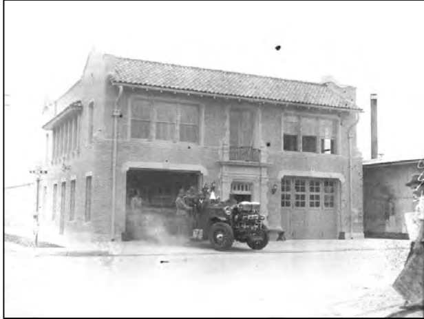
Figure 20: Fire Station No. 11 in 1925. Note red tile roof, bi-fold doors and roof drainage system. (ITC/San Antonio Light Collection)
