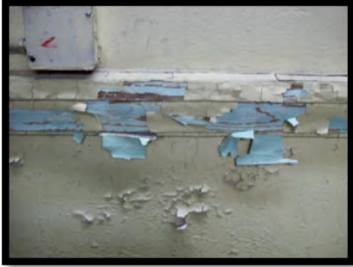
Figure 83: Paints and coatings applied to interior walls of Fire House No. 11 shall have VOC emissions not exceeding the VOC and chemical component limits of Green Seal Standards Requirements.
