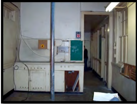
Figure 56: Fire pole can remain because it is a character defining feature, if there is a clearance of 32" for wheelchair to pass.
