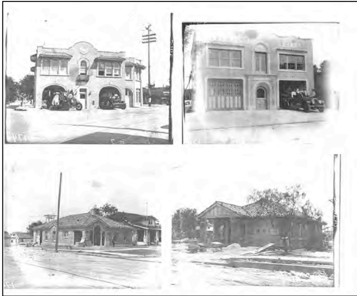
Figure 19: Fire Station No. 11 was constructed as part of a five-station building program; all five included the salient features of the Mission Revival/Spanish Colonial Revival style that was a popular choice for regional municipal buildings in 1920s Texas.
