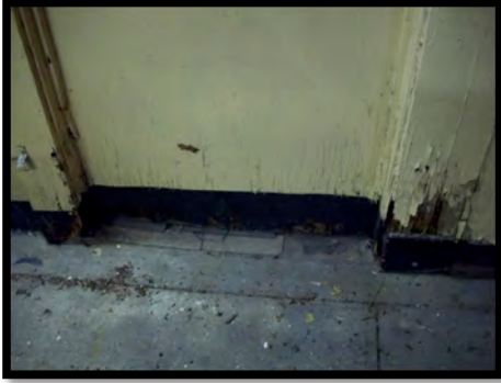
Figure 60: Floor shall be verified on site for any changes in level, for example from kitchen area towards left/right bay. The change in level shall be softened with a ramp.
