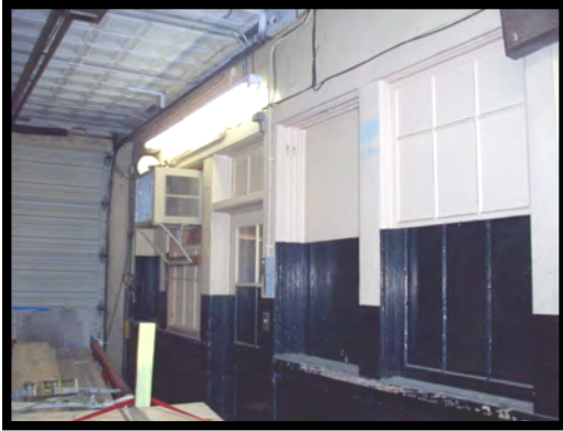
Figure 82: Increase natural ventilation by opening the garage doors during business hours or opening windows to allow for controlled airflow paths.
