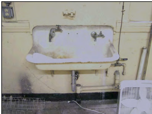
Figure 23: Cast iron sinks marked “Standard Sanitary Mfg. Co.” located in both apparatus bays are assumed to date from the first build, as well. (See Chronology of Development and Use for further information.)
