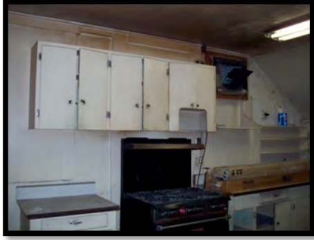
Figure 57: If cabinets are to be used by the public they shall be lowered to recommended height. Lower cabinets would require knee space for acceptable forward reach.
