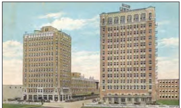
Figure 30: Nixon Office Building.
