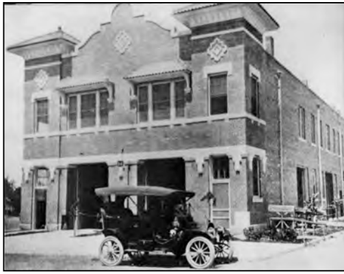
Figure 38: San Angelo City Hall and Fire Station (1912). (Fort Concho Museum)
