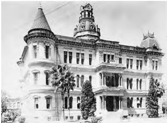
Figure 32: San Antonio City Hall, San Antonio, Texas. The before, left, and after, right, photos of the remodeling conducted in 1927. Tower and turret tops removed, fourth story with red tile roof added and major entrances extensively remodeled. (Historic American Building Survey)
