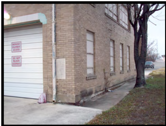
Figure 73: Sidewalks that will be reconstructed can use paving materials with a SRI of 29.
