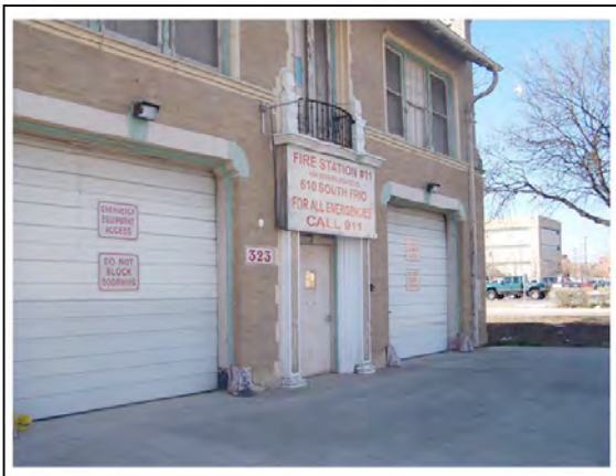
Figure 16: A temporary sign installed when the fire station was deactivated covered the upper door area for several years until removed in 2008. Current signage located on the bay doors indicates the historical use of the building as an active fire station.
