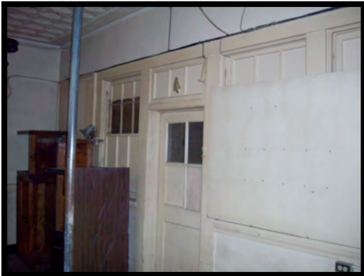
Figure 86: Remove paint on windows to allow a line of sight to the outdoor environment
