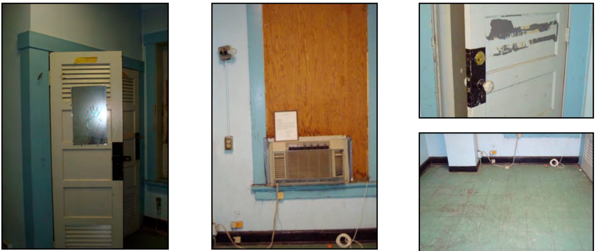
Figure 50: Offices; Similar Conditions in all Offices
