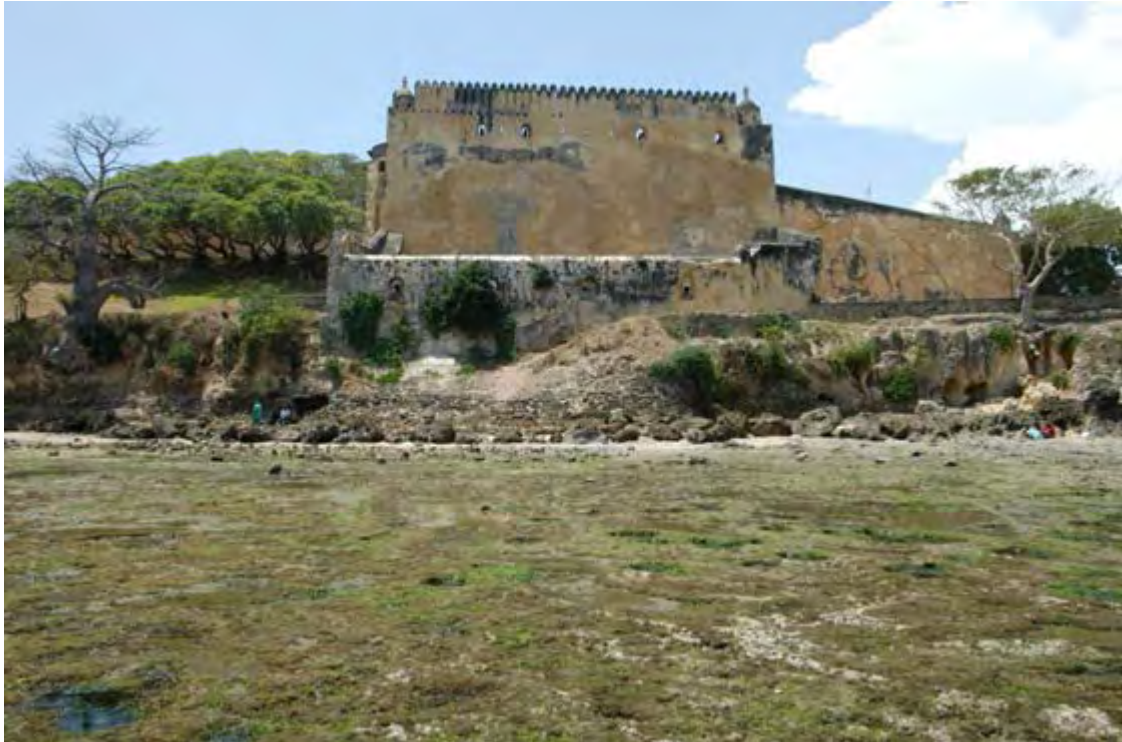
Figure 5. Effects of the tidal currents to the coral that forms the base of the Fort
