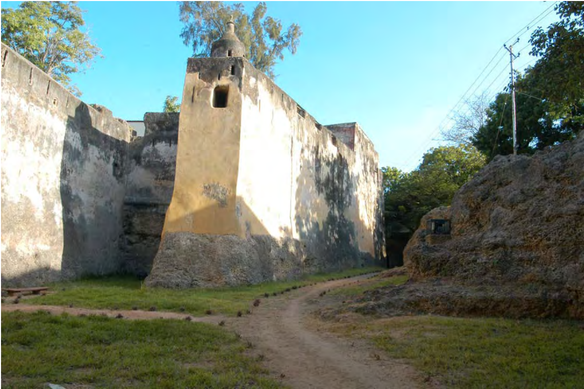
Figure 11. Moat of Fort Jesus, Mombasa
