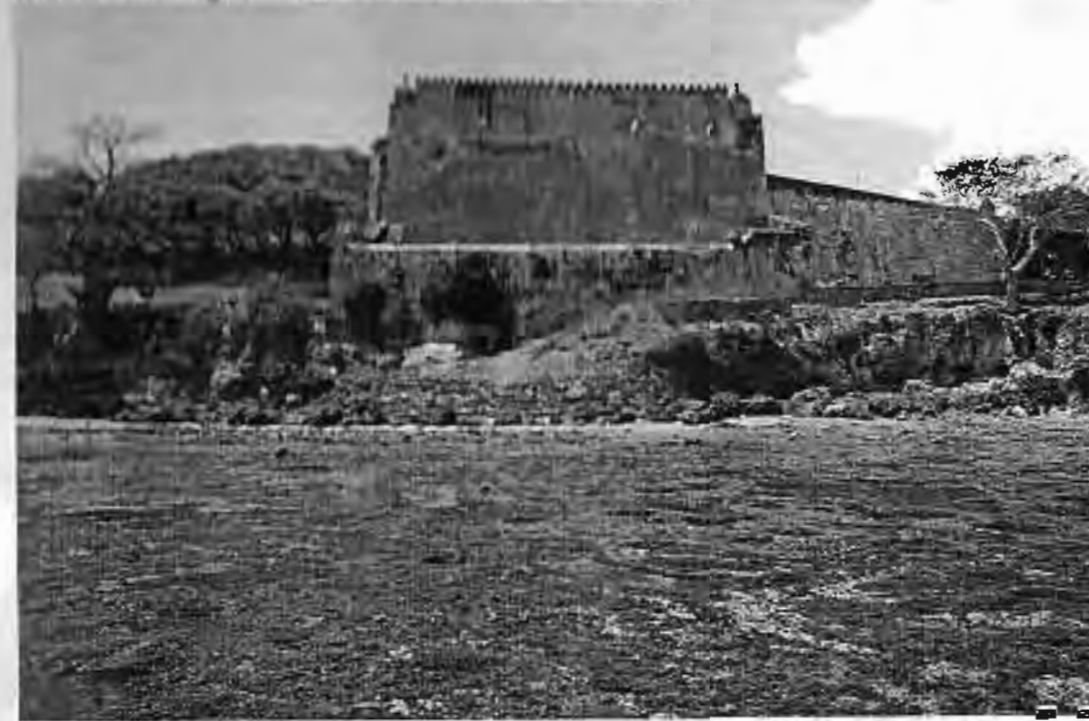
Figure 5. Effects of the tidal currents to the coral that forms the base of the Fort
