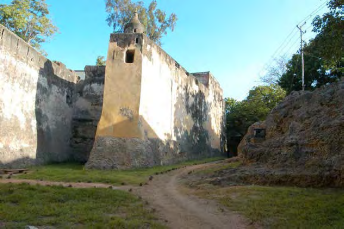
Figure 11. Moat of Fort Jesus, Mombasa
