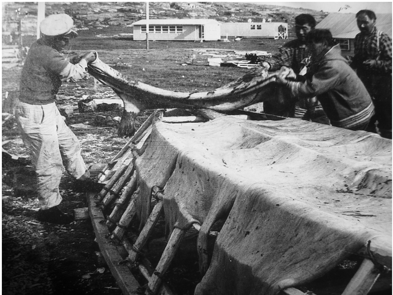
Figure 8. Building of a boat by fathers of interviewed elders in Ivujivik, 1960. Photo: Sarah and Mattiisi Iyaituk.
