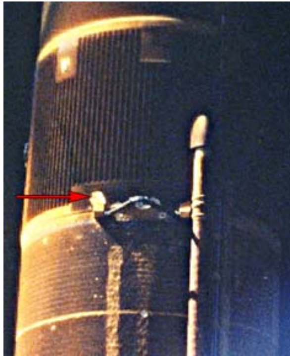
Figure 4.4.5.3 Image from STS-32 on-board umbilical well camera film showing damage to ET intertank TPS
