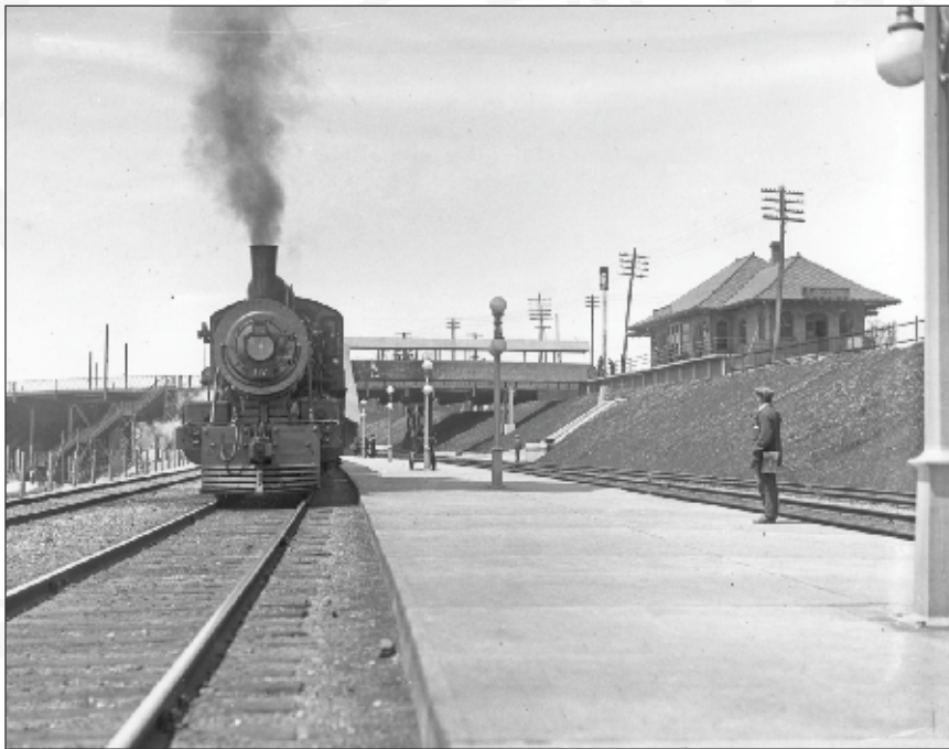
This 1915 view is looking west, Sunnyside Station is above the embankment on the right. The bridge beyond the station carried road traffic and streetcars down to Lakeshore Boulevard. The concrete portal on the embankment below the station led to an elevator for transporting baggage. The station was demolished in 1967 when GO Transit began operations. City of Toronto Archives, Fonds 1231, Item 1041.
