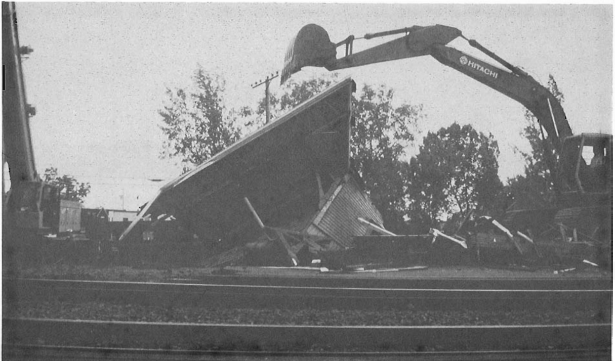
A sad end! The demolition of Val Royal station on June 5, 1995, less than three days after the end of service of the old CN electrics. Such was the end of a site beloved by railfans for many years.
