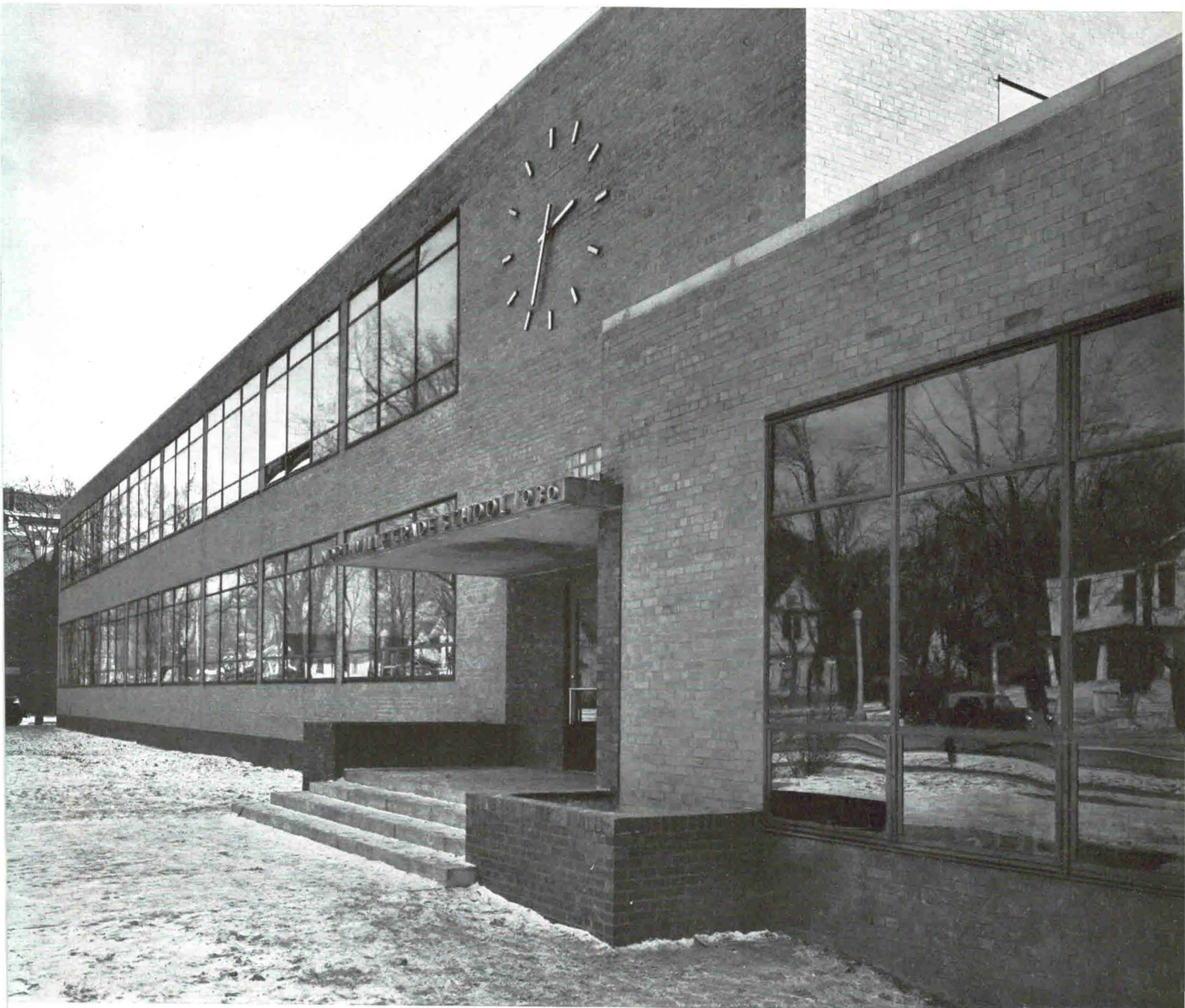
GRADE SCHOOL, NORTHVILLE, MICHIGAN LYNDON AND SMITH, ARCHITECTS
