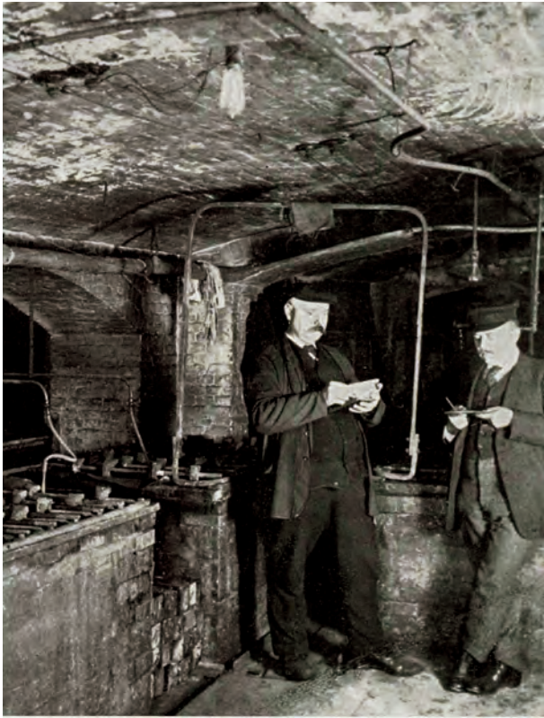
Copper tankhouse cells at Elbstrasse.
