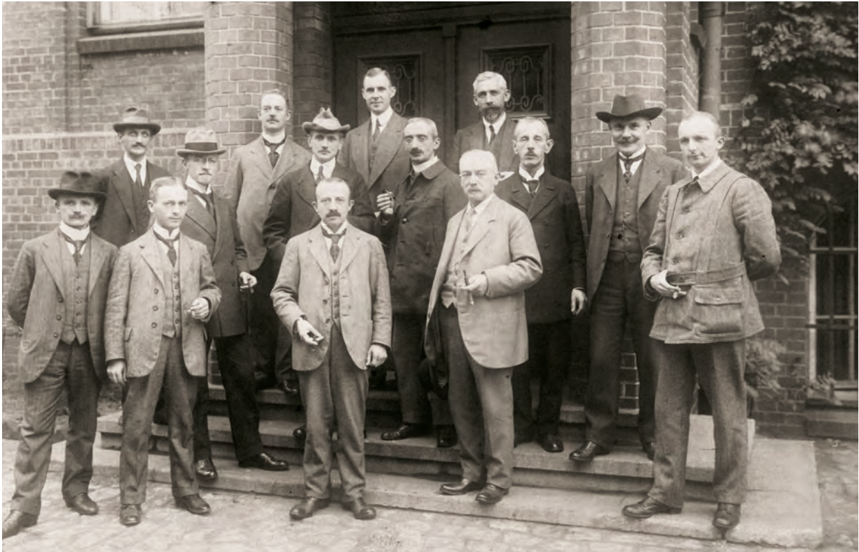
Management and staff members outside the entrance to the office building in 1917 (left to right). Top row: Messrs. Meyer, Hirsch (sales manager), Dr. Giuliani (copper tankhouse manager) and Herrgen. The central row shows Messrs. Lehmann, Dr. Tafel (technical director, 1914–1920), Dr. Wohlwill (Executive Board member, 1913–1933), Frank (authorized ore purchasing officer) and Baum (head of laboratory). Lined up in the front row are: Messrs. Lenk (successor of Baum), Dr. Stahl (chemical engineer), Nathansen (accounting), Schlesinger (Executive Board member, 1903–1924) and Hädrich (site manager).
