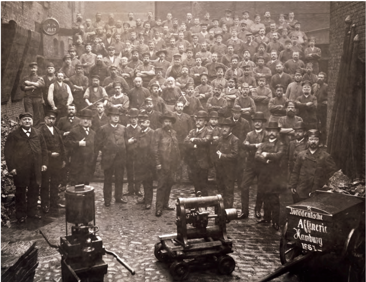
The workforce of NA in the yard of the Elbstrasse plant in 1887. In this year, approximately 200 employees produced almost 2,000 t of electrolytic copper.
