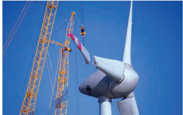
Everything revolves around copper: The generator of a modern wind power plant alone contains approximately 200 km of copper wire.
