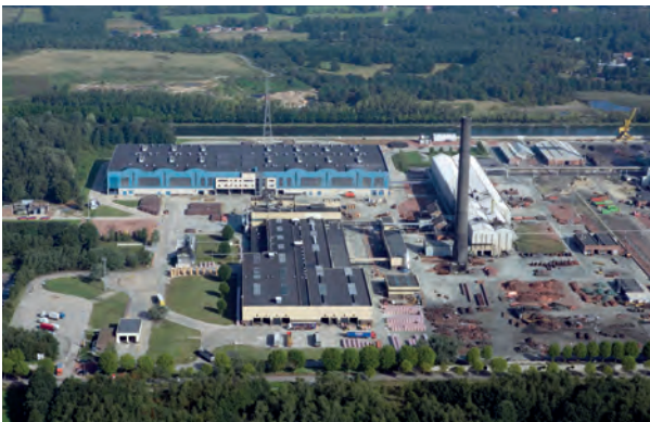
At Aurubis Belgium in Olen, approximately 30 km from Antwerp, about 500 employees produce anodes, cathodes, wire rod and specialty wire.
