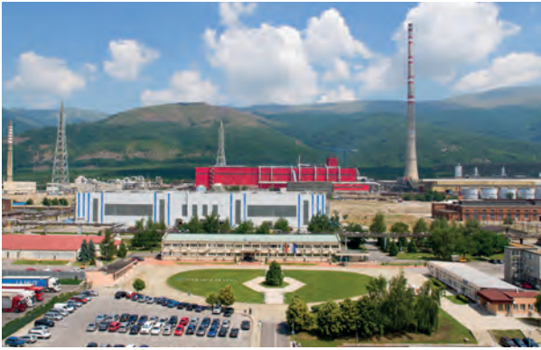
Aurubis Bulgaria in Pirdop is located about 90 km east of the capital city of Sofia. A new copper tankhouse was commissioned in Pirdop on October 28, 2008.
