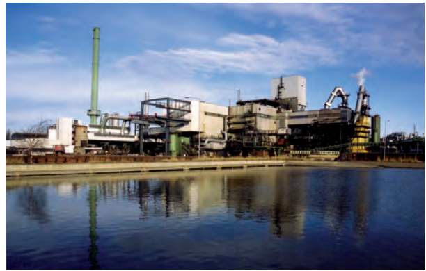
Fit for the future: the primary smelter (RWO), the centerpiece of unwrought copper production at Aurubis Hamburg, as it looks today. Time and again, the primary smelter was rebuilt and expanded, improved and honed.
