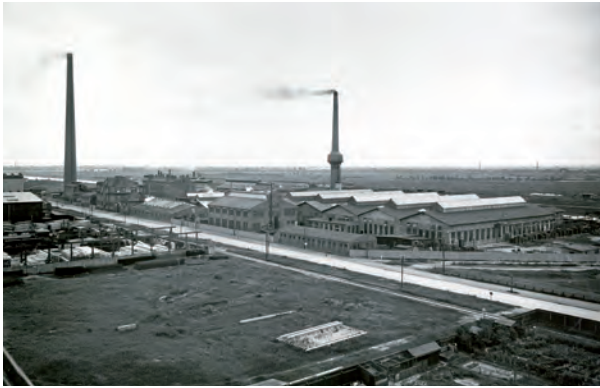
Several smokestacks were already in use in 1918, nearly 10 years after the move to Veddel Island.
