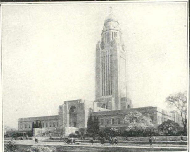
State Capitol at Lincoln, Nebr., is Athey-Shaded Crain, Goodhue & Ferguson, New York, Architects
