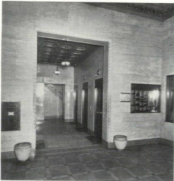
Remodeled Entrance and Elevator Lobby, Rose Building, Cleveland
