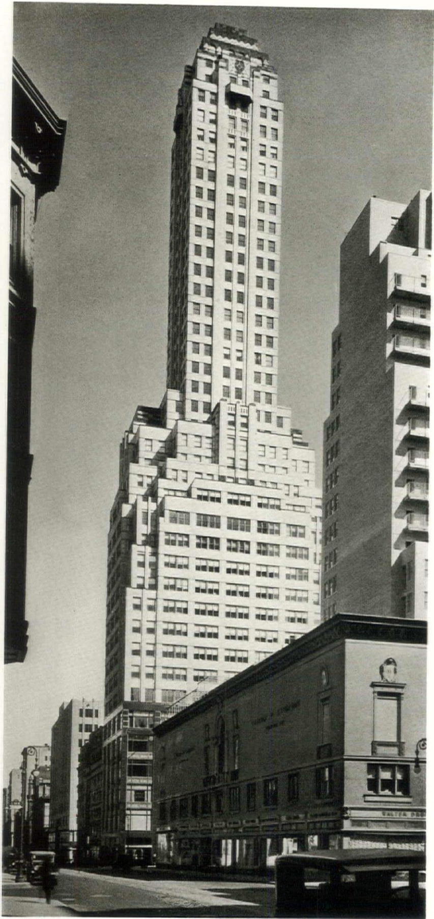
FULLER BUILDING, NEW YORK. WALKER & GILLETTE, ARCHITECTS
