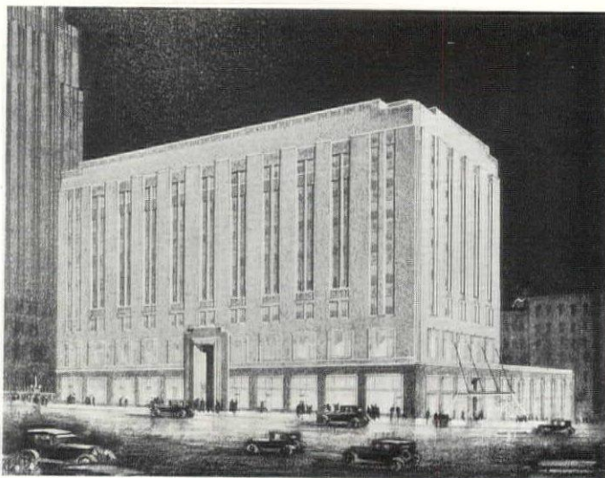
First Section as Built
