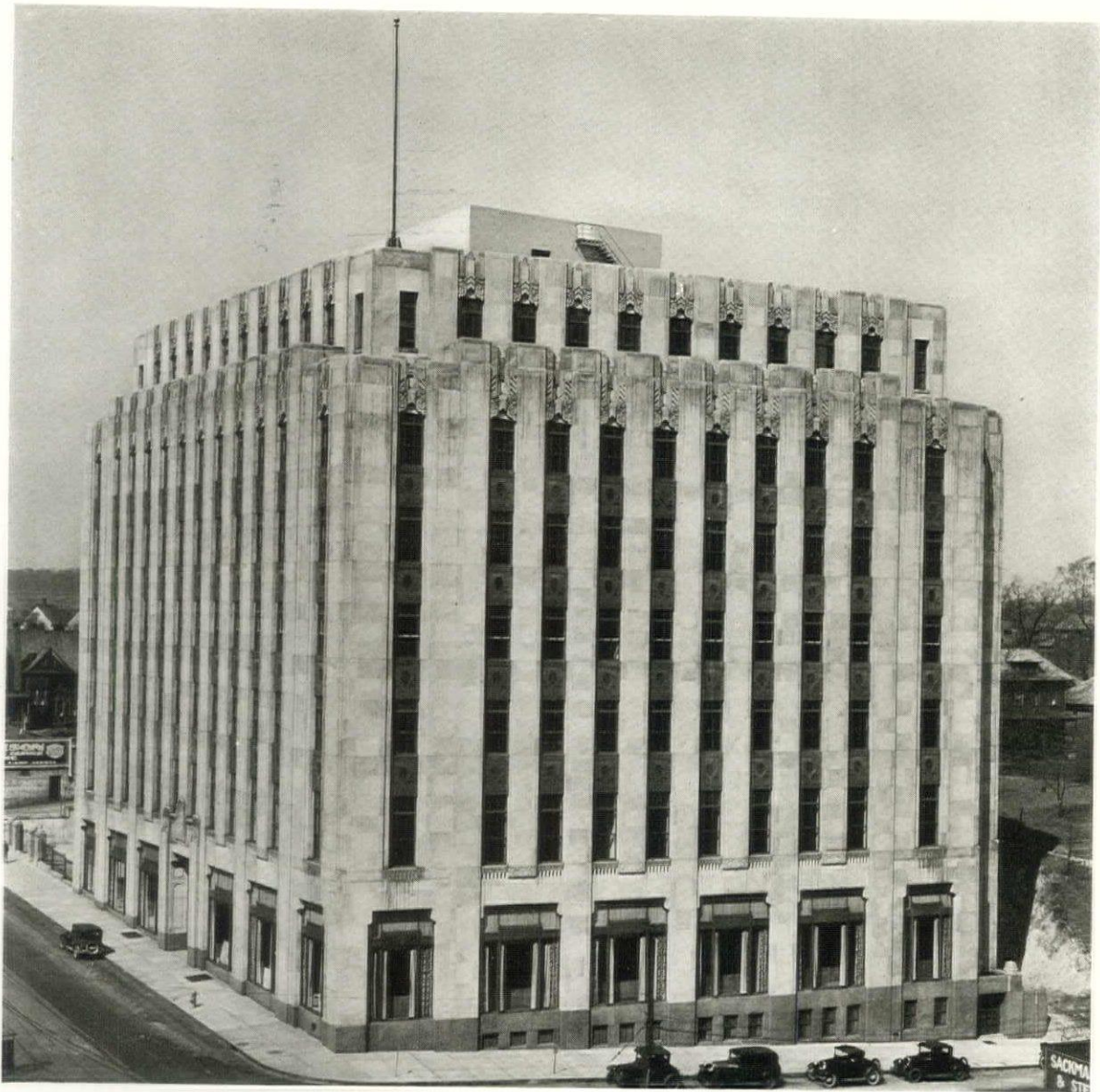
BUILDING FOR THE OHIO BELL TELEPHONE CO., AKRON. MILLS, RHINES, BELLMAN & NORDHOFF, INC., ARCHITECTS
