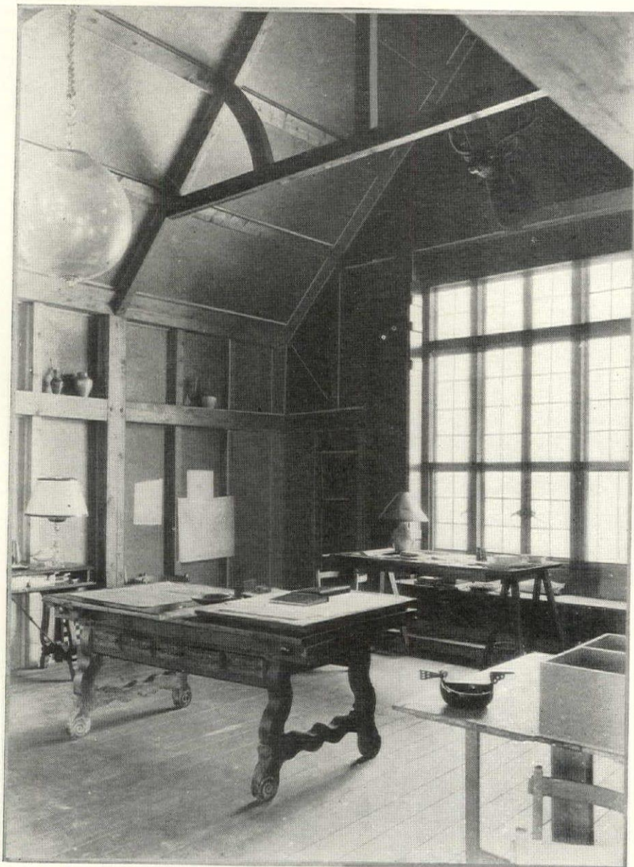
In Mrs. Archibald M. Brown's studio at Southampton, Long Island, the interior has been finished in heavy spruce timbers with Johns-Manville Insulating Board between. The architects were Peabody, Wilson & Brown.
