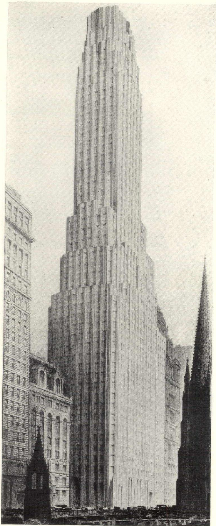
Irving Trust Company Building, being erected at One Wall Street, corner of Broadway, New York City. Voorhees, Gmelin & Walker, Architects. Marc Eidlitz & Son, Inc., Builders.
