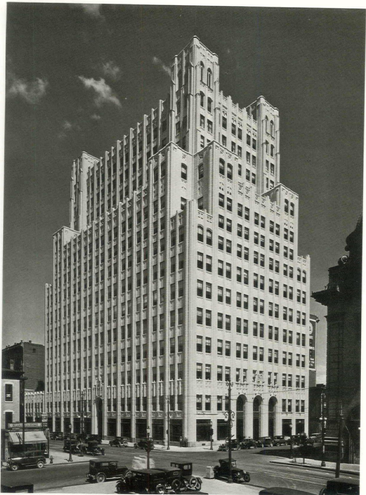
MOUNTAIN STATES TELEPHONE & TELEGRAPH BUILDING, DENVER. W. N. BOWMAN, INC., ARCHITECTS
