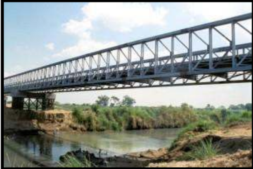
7: Line of Communication Bridge
