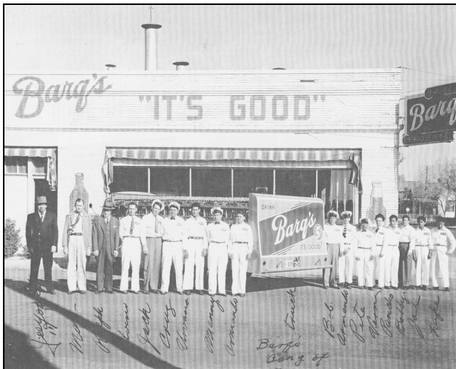
Figure 11b-6 – John Yowell and employees in front of the plant in 1947 (Courtesy of Dub Yowell)
