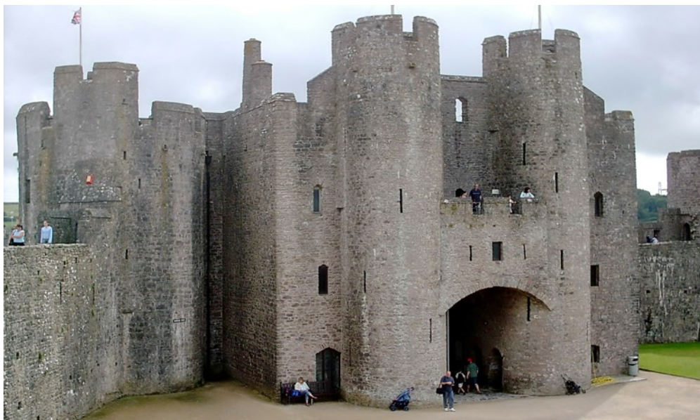
Fig. 42. Pembroke. Interior view of the Outer Gatehouse c. 1250, highlighting the mirrored and paired stair turrets either side of the (later) flying arch over the gatehouse passage.
