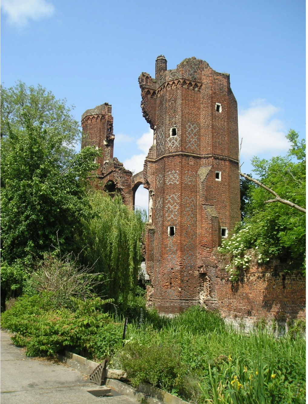
Fig. 70. Nether Hall (or Netherhall), Roydon Essex, c. 1460s. Remains of the gatehouse. An early example of a prestigious brick-built gatehouse tower. The remaining standing building is built of brick with blue brick diaper (an all-over surface decoration of a small repeated pattern) work and decorated with trefoiled corbel friezes. The single ACW staircase turret is to the right, with the decorative corbelling. Built by Thomas Colte, the richest commoner of Edward V's regime, it is one of the most accomplished fifteenth century works of brick architecture anywhere in England.
