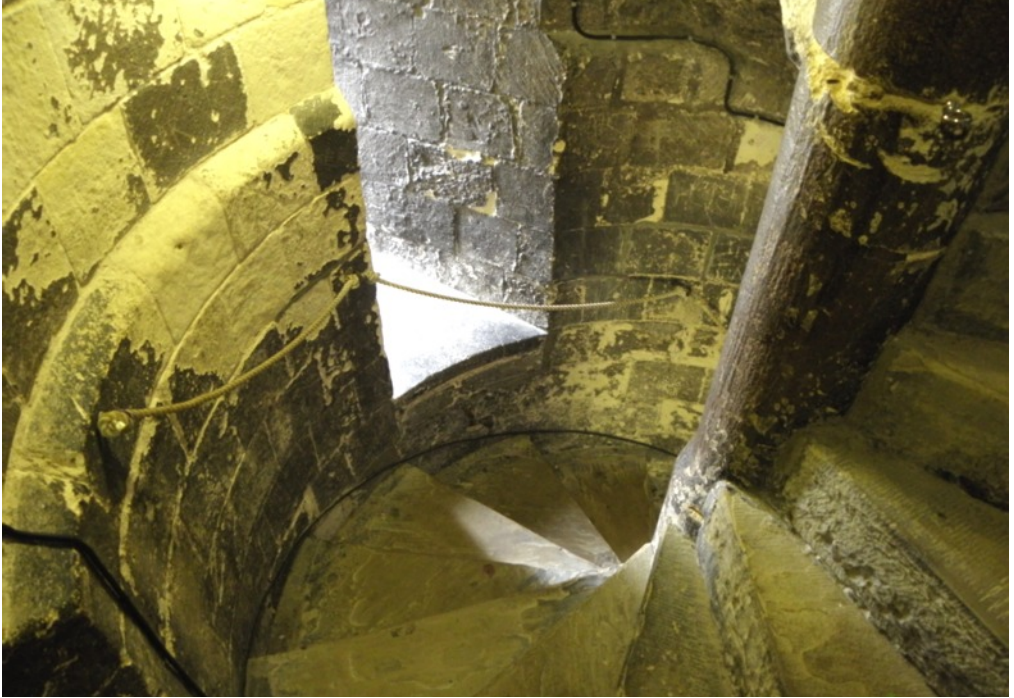
Fig. 10. Norwich Castle. ACW anticlockwise stair in the NE corner buttress. As seen here, the solid newel drums reduce in diameter when the spiral reaches the first floor level (fifth stair from top right).
