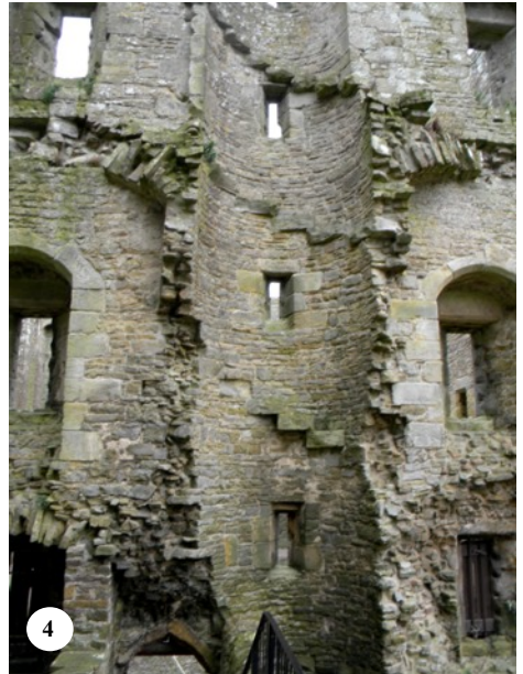
Fig. 66. Bolton Castle ACW stairs. 1. SW stairs, entry up to chapel and lodgings. 2. SW stairs looking down from the first floor. 3. SW Stairs from the ground floor. 4. East (Gateway entrance) range, remains of spacious centrally-placed stair up to lodgings at either side.
