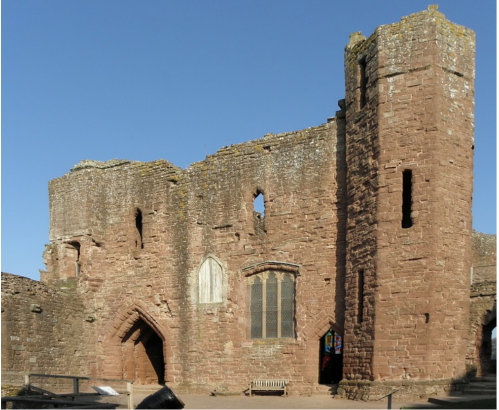
Fig. 48. Goodrich Castle. Rear of the gatehouse with the octagonal stair turret (right), c. 1310-20 (Stair width 1.25m; tread/ riser height 18.4 cms ). Figs. 49, 50. Below. The octagonal stair turret with CW cut-slab winders c. 1300-10.
