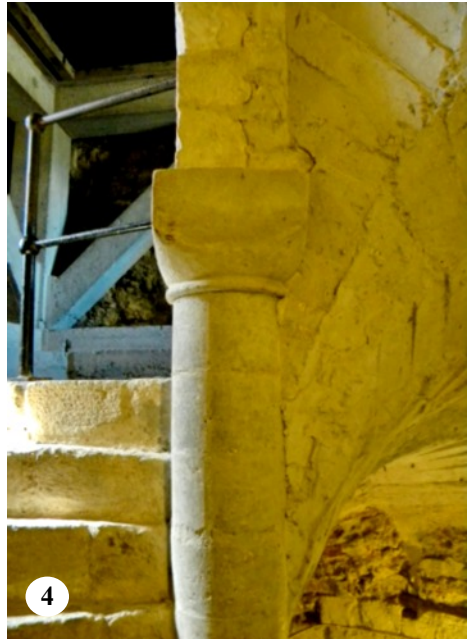
Fig. 33. 1: Colchester Great Tower - 1070s - CW (an 1890s print). 2: Rochester - 1130s, CW, NE turret, first floor. The newels have been robbed.. 3: Hedingham Great Tower - 1140s - CW. Original stone steps have been replaced by brick. 4: Orford Castle, 1160s, CW stair, at the top of the spiral with capital and centering imprints to the right.
