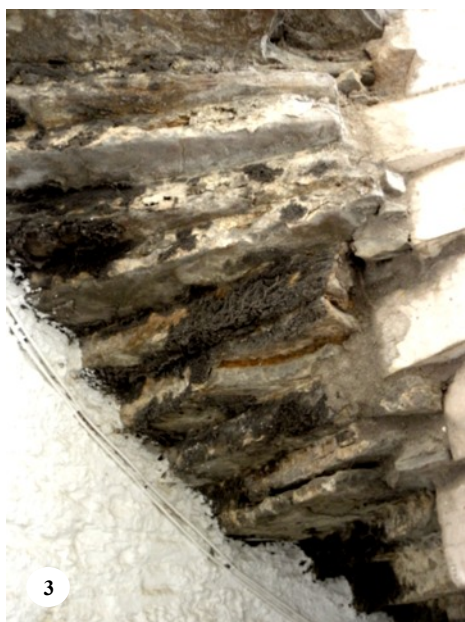
Fig. 47. Caerphilly Castle. 1. Inner East Gate house. The north ACW stair turret - ground floor (with renewed newels). Width 1.48m. 2. Inner East Gatehouse, north ACW stair turret (with renewed newels) first floor. Winder width 1.48m. 3. Inner East Gatehouse - north ACW stair turret (with renewed newels) first floor, highlighting the original winders embedded into the turret casing (2 overlaid cut-slabs per winder). 4. Remains of the destroyed NE Tower of the Inner Ward with its ACW stair.
