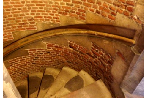
Fig. 73. Tattershall Castle. c. 1440s. CW stairs, with stone cut-slabs and ashlar hand-rail. Detail of the hand-rail.
