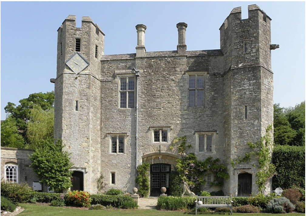
Fig. 58. Above: Boarstall Tower gatehouse, c. 1312-14. Central bay over entrance, balusters, chimney stacks, later. The original gatehouse to a country seat, now lost. Fig 59. Below: Boarstall Tower. Rear (south) view. \frac{3}{4} round hexagonal stair turrets with independent ground-floor doors in the courtyard. These rear doors to the turrets were originally the only access to the upper floor(s). The pattern of fenestration (though not the present style - they are early C17) is similar to Caerphilly and Tonbridge. The interior of the turrets are cylindrical. The east turret (right) is larger than the west; tread width 0.92m. Arrow loops are similar to the Kenilworth Water Tower.
