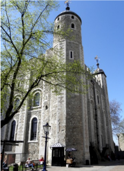
Fig. 4. The White Tower, c. 1070-1100. The principal NE staircase turret - appearing polygonal to the lower exterior and circular to the top.
