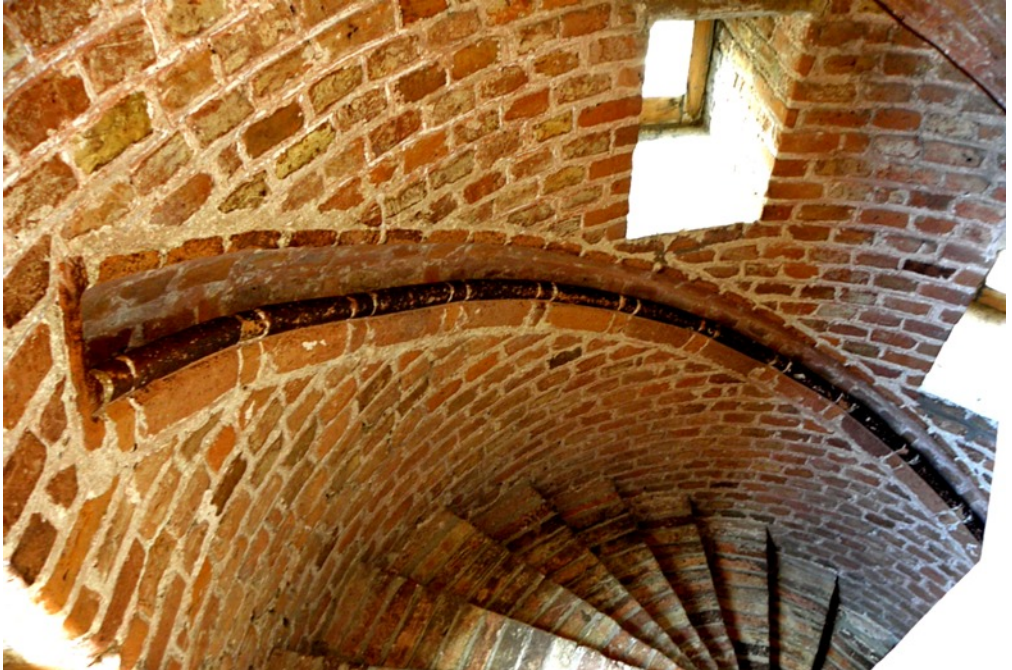
Fig. 71. Oxburgh Hall. c. 1480s. West gatehouse turret. ACW stairs, not matched or mirrored in the east turret. Brick newels, winders, countersunk handrail and vaulting.
