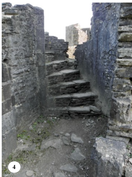
Fig. 47. Caerphilly Castle. 1. Inner East Gate house. The north ACW stair turret - ground floor (with renewed newels). Width 1.48m. 2. Inner East Gatehouse, north ACW stair turret (with renewed newels) first floor. Winder width 1.48m. 3. Inner East Gatehouse - north ACW stair turret (with renewed newels) first floor, highlighting the original winders embedded into the turret casing (2 overlaid cut-slabs per winder). 4. Remains of the destroyed NE Tower of the Inner Ward with its ACW stair.
