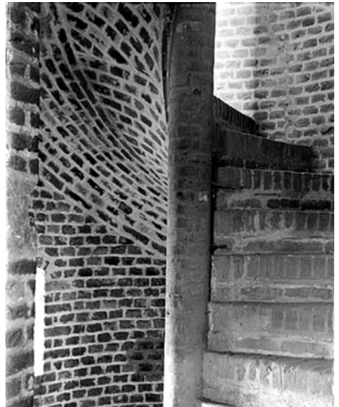
Fig. 82. Faulkbourne Hall. c. 1480-90s. 3/4-octagonal ACW stair turret with brick vaulting, on the corner of the lodging tower, and entered from within the tower. Image from Nathaniel Lloyd's 'A History of English Brickwork' 1925, p. 371. Probably contemporary with Oxburgh, and constructed by the same workmen. See also Gomme and Maguire, 2008, p. 99, who considered that the tower was a late design change in the course of construction.
