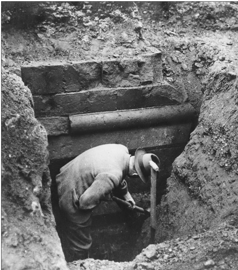
Fig. 20. Above. Brandon Castle. A previously unpublished photograph of the excavation of Brandon castle in 1948. In the picture the excavator, John Edwards, is seen in front of the buttressed W corner of the tower. The stonework is beautifully worked ashlar and some of the pieces are truly monolithic. The mouldings of the plinth are comparable with Bamburgh (1130s). Working on site at the time was a youthful Anthony Emery who arranged for this picture to be taken, and in whose archive it remains. The image is reproduced courtesy of and ©Anthony Emery.
