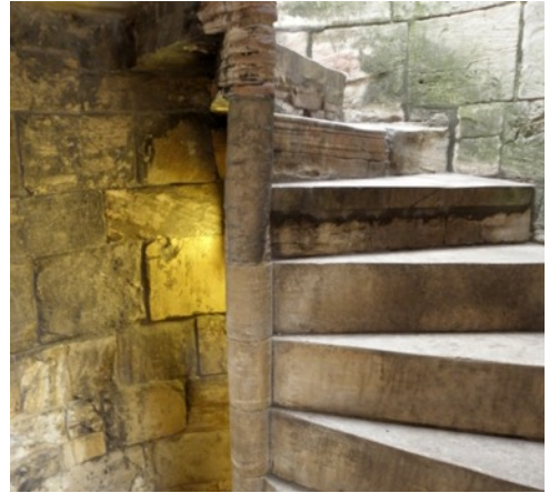
Fig. 40. Above. Clifford's Tower - York. North ACW stairs. One-piece newel and winder. Many of the step's tops have been replaced/resurfaced. Tread height 20 cms. Fig. 41. Below: The ACW stair from the wall-walk.
