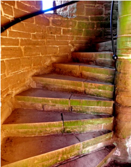
Fig. 48. Goodrich Castle. Rear of the gatehouse with the octagonal stair turret (right), c. 1310-20 (Stair width 1.25m; tread/ riser height 18.4 cms ). Figs. 49, 50. Below. The octagonal stair turret with CW cut-slab winders c. 1300-10.
