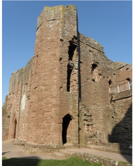
Fig. 48. Goodrich Castle. Rear of the gatehouse with the octagonal stair turret (right), c. 1310-20 (Stair width 1.25m; tread/ riser height 18.4 cms ). Figs. 49, 50. Below. The octagonal stair turret with CW cut-slab winders c. 1300-10.
