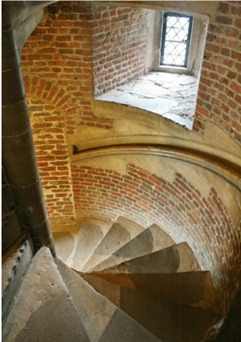
Fig. 72. Tattershall Castle. c. 1440s. CW stairs, with stone cut-slabs and ashlar hand-rail.
