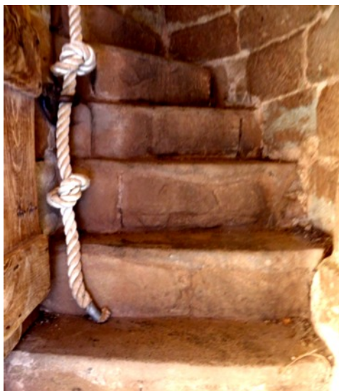
Fig. 26. Goodrich Castle. The start of the vaulted ACW stair in the NW corner buttress.
