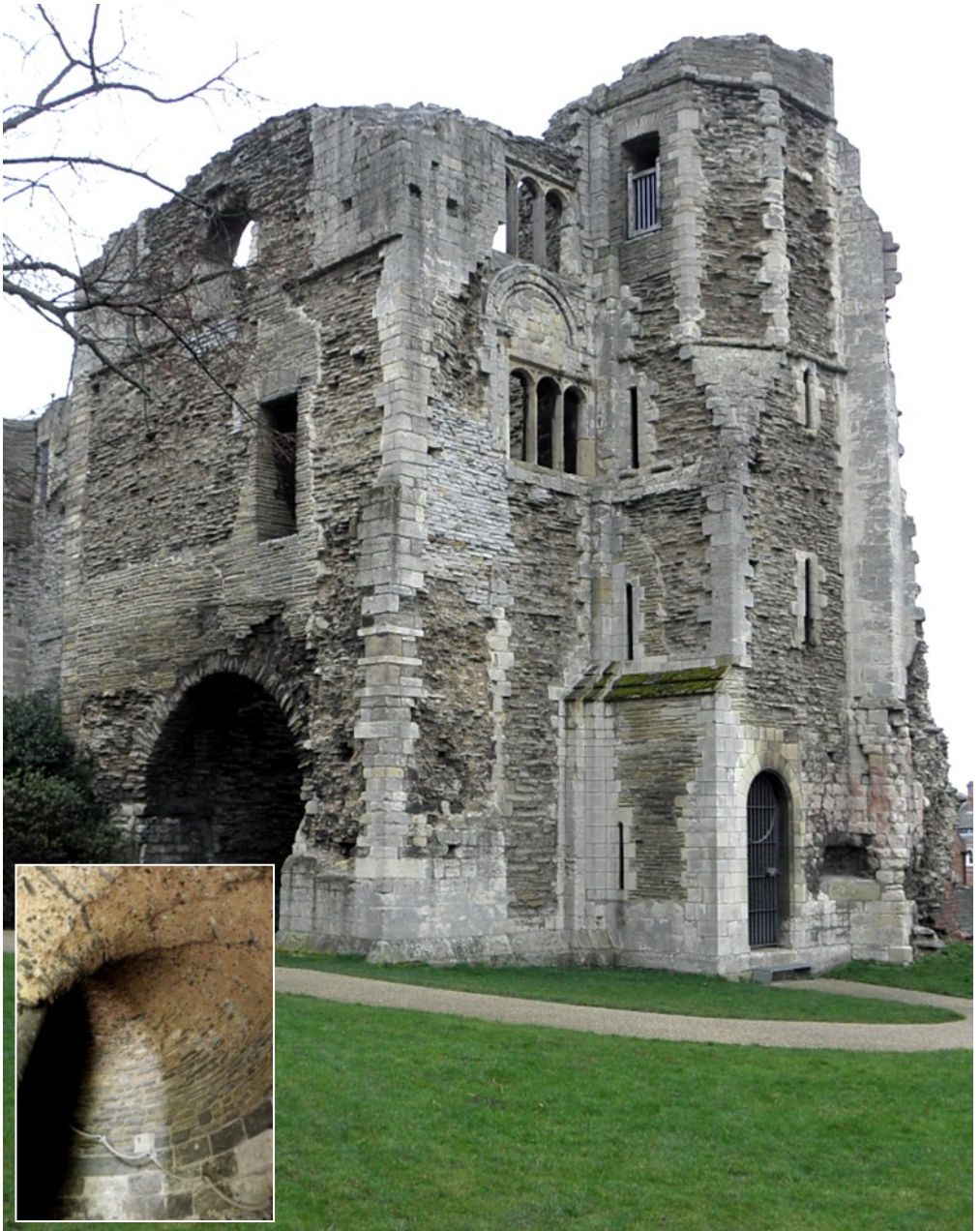
Figs. 14 & 15. Newark on Trent. The south and eastern façades of the 1130-40s gatehouse, showing the integral staircase turret, with its (rebuilt and re-faced post-1900) ground-floor entrance, giving access to a palatial audience chamber directly over the entrance passage, and access to the demolished eastern wall walk at the top. Unusually, the staircase winds ACW. The current east entrance and immediate stonework on its south side is post-1900, and the stair-turret entrance may well have been to the south originally, with the south wall-face running vertically straight to the ground without the final outward offset. See the Francis Frith photographs: 24651, 24650 - Fig 13, 35553 and 35552. Inset: Fig. 15. A section of the vaulted roof of the Newark spiral, showing the gradual segments of vaulting with the impressions left by the progression of the timber centering.
