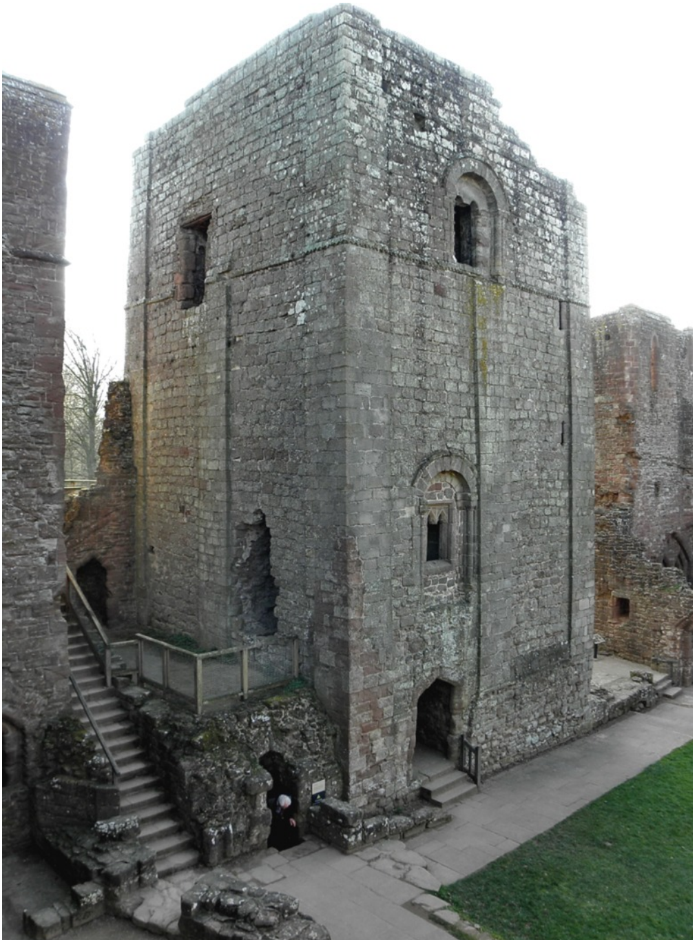
Fig. 27. Goodrich Castle, the donjon c. 1148-52. The ACW spiral starts on the first floor - at the level of the converted north-facing doorway (into a window) above the present basement entrance, and continues to the top in one continuous run. The two loops on the right of the tower near the clasping corner buttress indicate its location.
