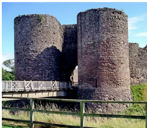
Fig. 35. White Castle, gatehouse, c. 1220-30s. With CW and ACW concentric mural stairs.
