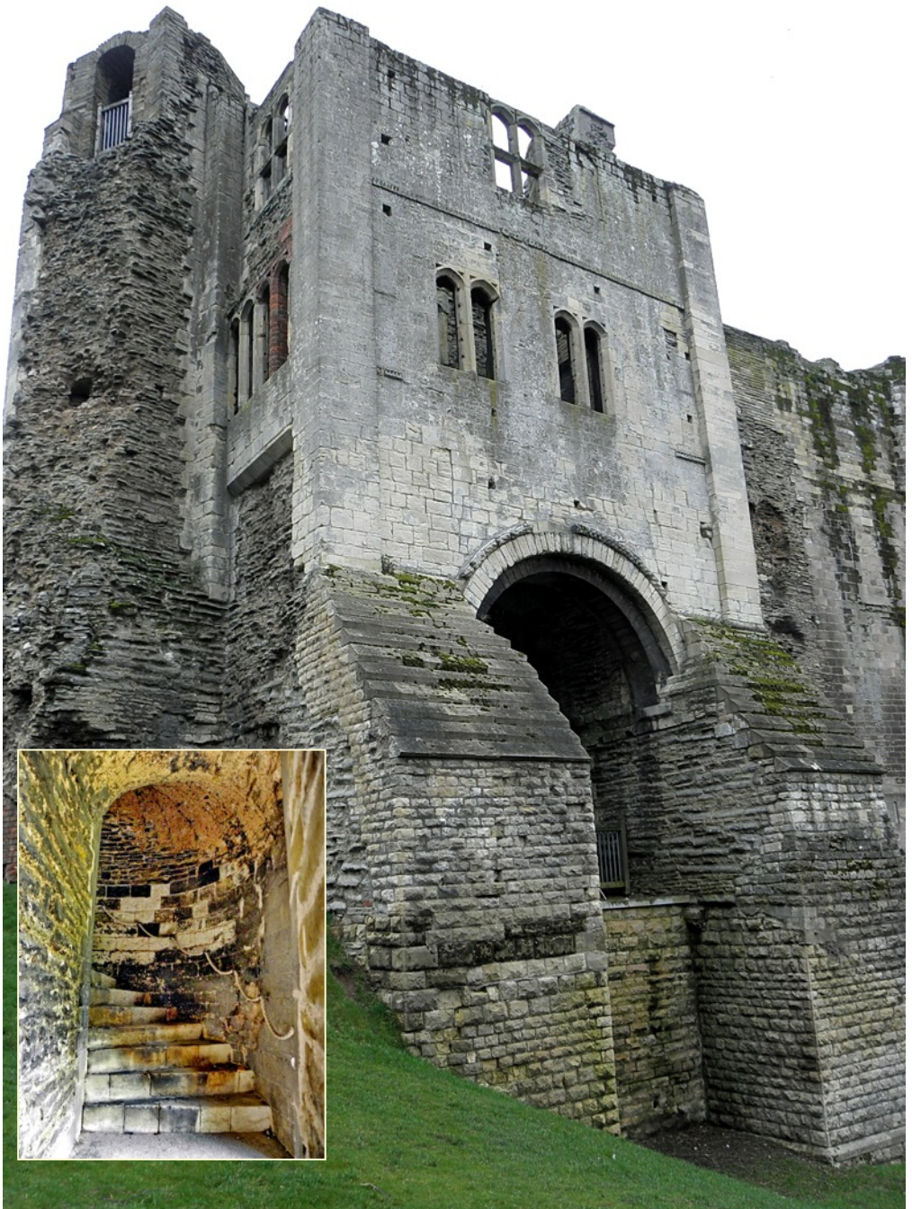
Figs. 16 & 17. North, entrance façade to the Newark gatehouse, with the stair turret to its left. Windows are later insertions. Below, left: Fig 17, Inset: The wide ACW spiral stairs, 1.57 metres width, the winders (part renewed stone) resting on vaulting and butting up to the newel- not part of it. The newel consists of stacked single-piece ashlar drums (like Norwich).
