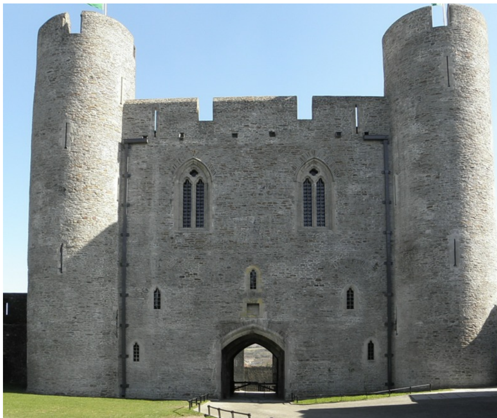
Fig 44. Caerphilly Castle. Inner East Gatehouse, 1268-71. The single room with the two large windows was probably the Constable's Hall. Note that, like Tonbridge, the stair turrets are not accessible from the inner ward.
