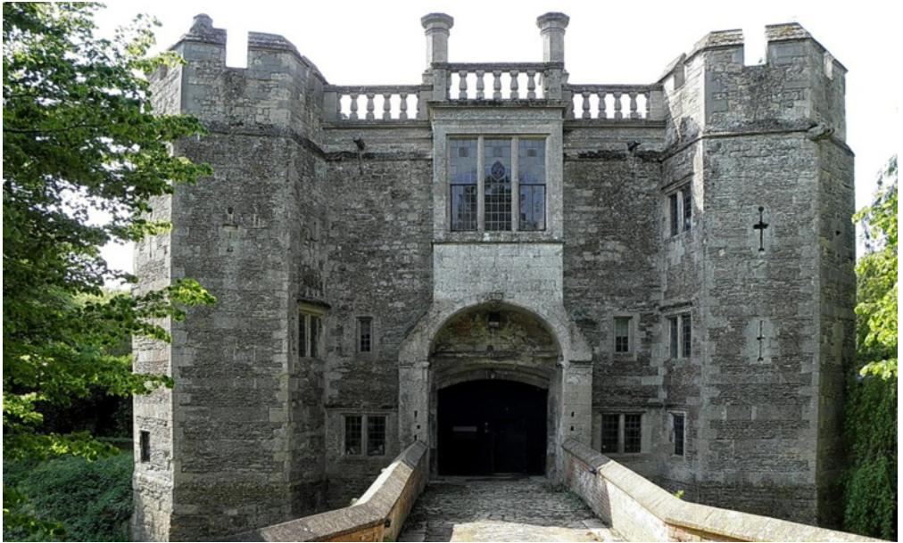
Fig. 58. Above: Boarstall Tower gatehouse, c. 1312-14. Central bay over entrance, balusters, chimney stacks, later. The original gatehouse to a country seat, now lost. Fig 59. Below: Boarstall Tower. Rear (south) view. \frac{3}{4} round hexagonal stair turrets with independent ground-floor doors in the courtyard. These rear doors to the turrets were originally the only access to the upper floor(s). The pattern of fenestration (though not the present style - they are early C17) is similar to Caerphilly and Tonbridge. The interior of the turrets are cylindrical. The east turret (right) is larger than the west; tread width 0.92m. Arrow loops are similar to the Kenilworth Water Tower.
