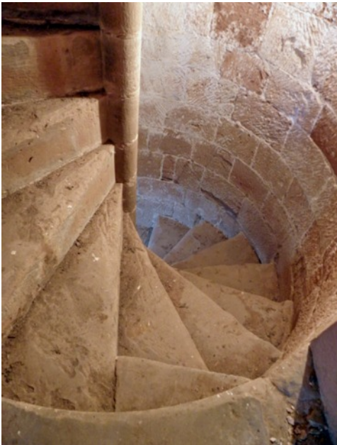
Fig 62. Above. Maxstoke Castle. First floor 'Constable's Chamber' over the gatehouse passage, looking towards the west window (right) and south window (left), and door to the wall-walk. Fig. 63. Below left. The SE stair turret looking down from the first floor. Fig 64. Below right. The smoothed sculptural undersides of the cut-slabs producing a seamless curvaceous helix.
