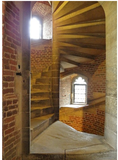
Fig. 74. Tattershall Castle. c. 1440s. CW stairs, with stone cut-slab winders and ashlar hand-rail.
