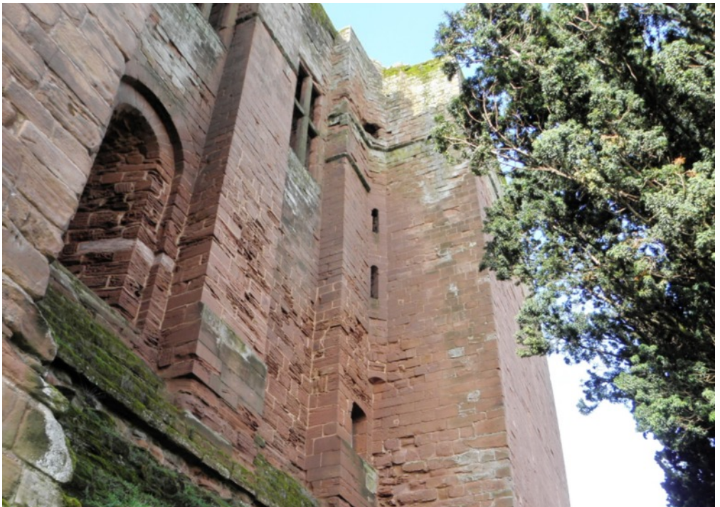
Fig 22. Above: Kenilworth Castle. The great tower, c. 1125-30, from the south. Fig. 23. Below: The great tower from the east. The NE staircase turret to the north (right). Small slit loops in the chamfered angle lit the spiral stair.
