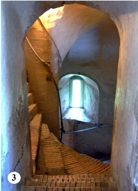
Fig. 33. 1: Colchester Great Tower - 1070s - CW (an 1890s print). 2: Rochester - 1130s, CW, NE turret, first floor. The newels have been robbed.. 3: Hedingham Great Tower - 1140s - CW. Original stone steps have been replaced by brick. 4: Orford Castle, 1160s, CW stair, at the top of the spiral with capital and centering imprints to the right.
