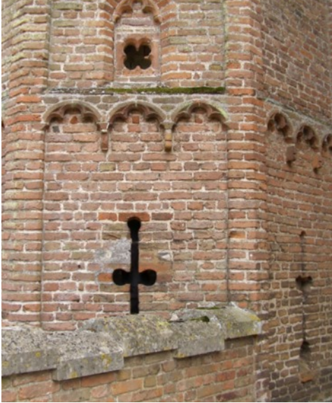
Fig. 80. Oxburgh Hall c. 1482. Decorative arrow loops in the east gatehouse turret.
