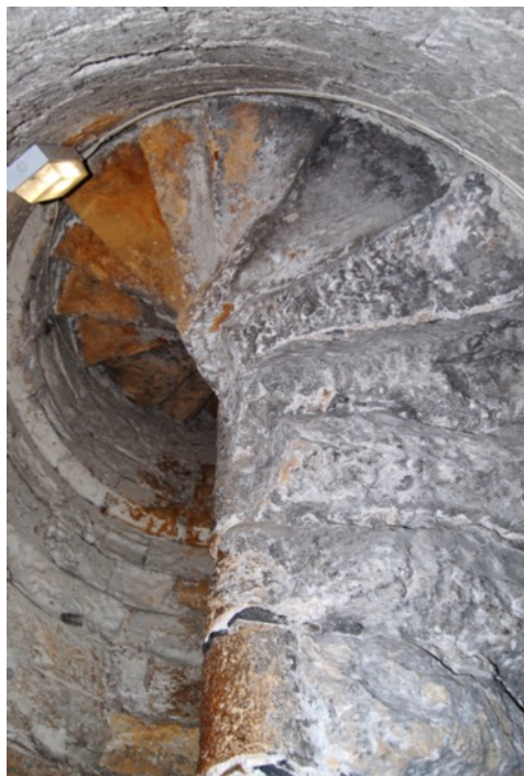
Fig. 82. Carrickfergus Castle, Ulster, c. 1180-90s. The rough underside of the earliest known one-piece cut-slab spiral stair in the British Isles.
