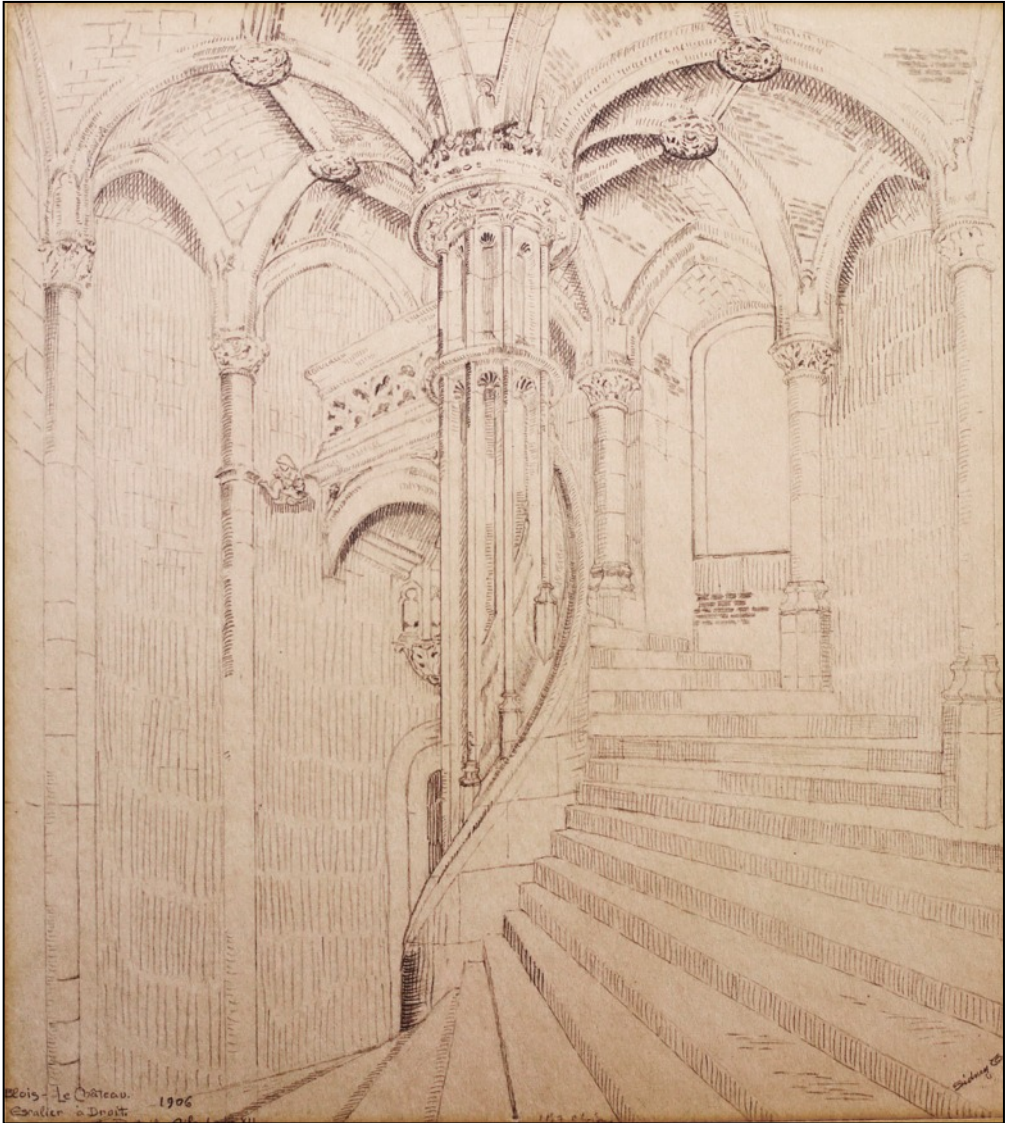
Fig. 89. Château Blois. Not the Renaissance stair, but a late-medieval anticlockwise stair in the Louis XII wing of the same building. Drawing by Sidney Toy, 1906, marked 'Escalier à Droite'. Built at the very end of the 15th century. Reproduced by courtesy of Sidney Toy's family.
