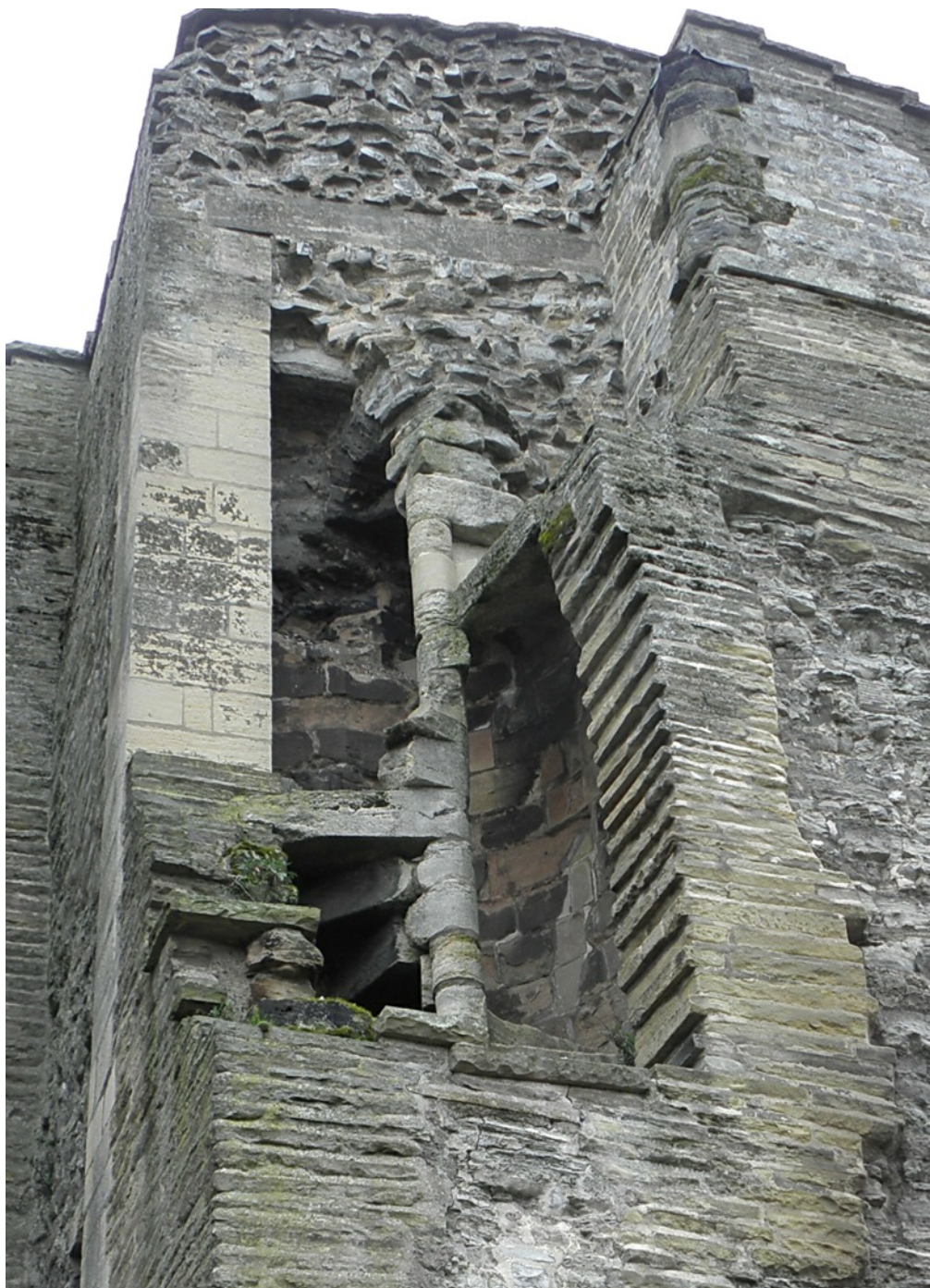
Fig. 53. Newark on Trent Castle. West curtain c. 1300-1310. Anticlockwise ascending stairs adjacent to the Middle Tower, rising from a window recess in the Great Hall. It can be readily observed that the steps (winders and newels) are one solid cut-slab piece and that the winder ends dovetail quite deeply into the face of the cylinder shaft or turret
