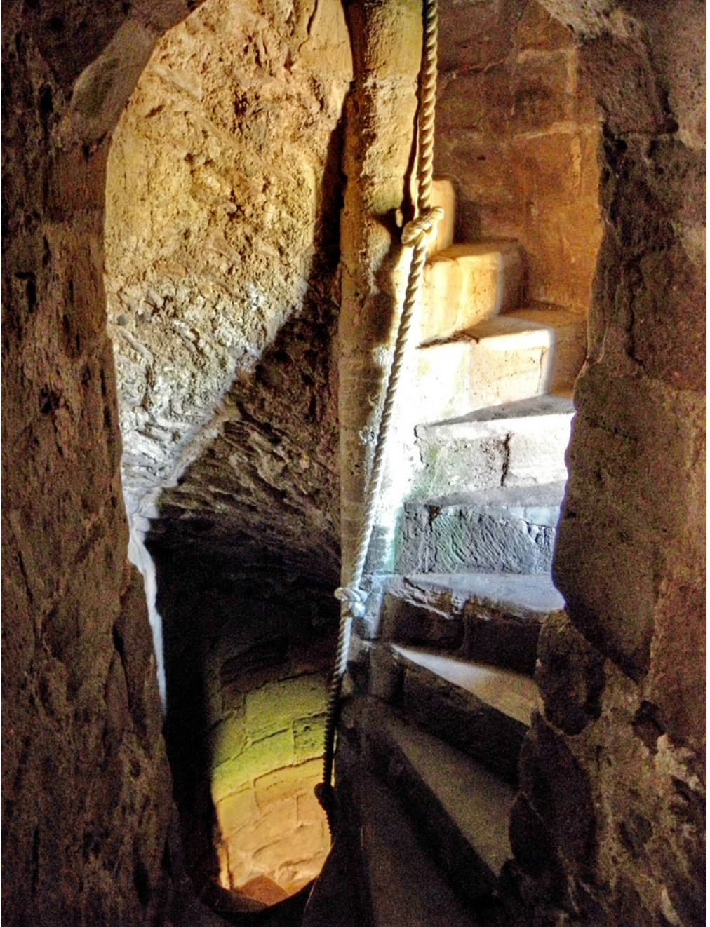
Fig. 28. Goodrich Castle. The Norman donjon, c. 1148-52. The precipitous spiral stair in the NW corner buttress, rising from the first floor to the roof. Vaulted, with steeply rising treads. Riser height 21 cms (8.5 in.), tread width 0.7m. (cf. Colchester 2.15m). Whilst current UK building regulations allow a riser height of between 17 and 22 cms, the regulations recommend builders should stay ideally between a range between 19 and 21 cms to build a flight that is most comfortable in use. (Building Regulations 2000, Section 1, Stairs and Ladders, Part K, K1, paras 1.1-1.6)
