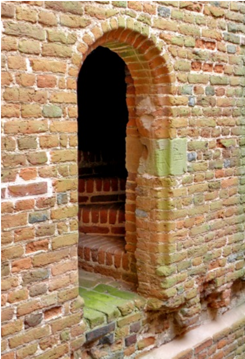
Fig. 78. Kirby Muxloe Castle, c. 1480-83. West Tower. ACW room stairs rising to the latrines at each floor level. Tread widths: 1.08m. Riser height: 21 cms.
