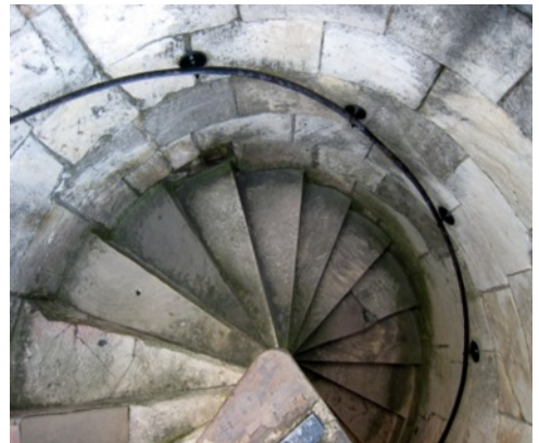
Fig. 40. Above. Clifford's Tower - York. North ACW stairs. One-piece newel and winder. Many of the step's tops have been replaced/resurfaced. Tread height 20 cms. Fig. 41. Below: The ACW stair from the wall-walk.
