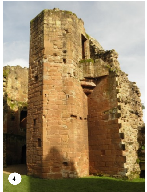
Fig. 54. 1: Kenilworth, Lunn's Tower (1210-15) from the west. 2: Lunn's Tower floor plans, © & courtesy English Heritage (EH Guidebook p. 31). 3: The added c. 1310-14? ACW cut-slab staircase in the semi-octagonal stair-turret seen above in (1) and (4). Winder width 0.82m, height 23cms). 4: View of the Lunn's Tower staircase turret from the SW, located outside the perimeter curve of the tower, enabling the tower chambers to be used as private accommodation.
