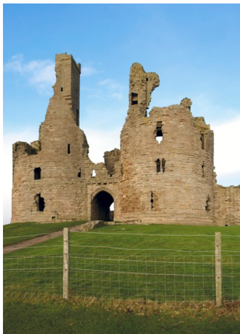
Fig. 51. Dunstanburgh. Gatehouse c. 1314-20 from the south, with mirrored CW (east, right) and ACW spiral stairs (west, left) within the wall thickness.
