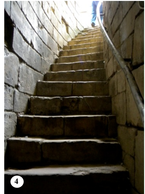
Fig. 34. 1: Scarborough Castle - 1160s - CW, stairs from the basement located in the middle of the wall. 2 Middleham Castle - 1170s - CW. 3: Dover Castle - 1180s - vaulted CW stairs - NE . 4: Conisbrough - 1190s - Mural CW.
