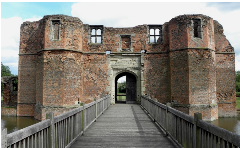
Fig. 75. Kirby Muxloe Castle, c. 1480-83. The entrance façade from the north-west. The Licence to Crenellate was issued in 1474. The gatehouse is extensively decorated with diaper work under the direction of John Cowper, master-mason. Fig. 76. Below: The south-west-facing courtyard façade of the gatehouse. Symmetry is evident with mirrored pairs of staircase turrets accessed from the stone-surround doors in each turret. The ACW stair is in the right (NE) turret.
