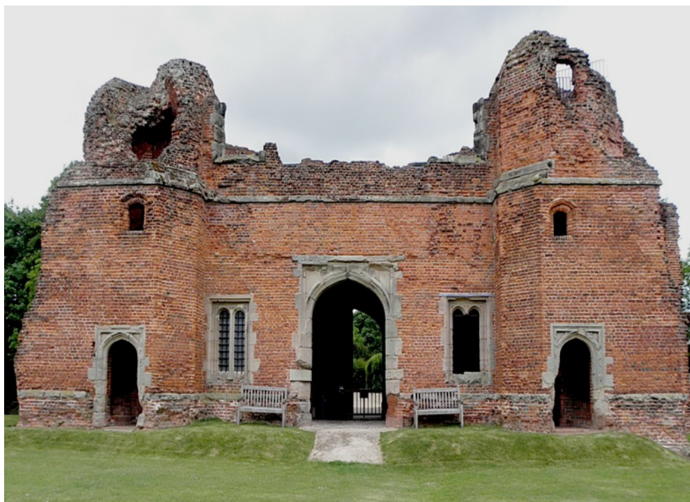
Fig. 75. Kirby Muxloe Castle, c. 1480-83. The entrance façade from the north-west. The Licence to Crenellate was issued in 1474. The gatehouse is extensively decorated with diaper work under the direction of John Cowper, master-mason. Fig. 76. Below: The south-west-facing courtyard façade of the gatehouse. Symmetry is evident with mirrored pairs of staircase turrets accessed from the stone-surround doors in each turret. The ACW stair is in the right (NE) turret.
