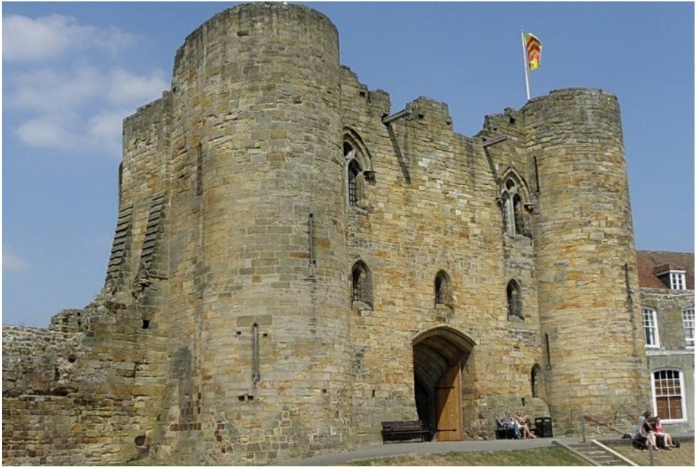
Fig. 43. Tonbridge. c. 1250-60s. The gatehouse from the bailey, with the the half-round stair turrets at the angles. A four storey self-contained block of outstanding virtuoso quality. Tread risers are a monumental 28+cms and are probably the steepest stair treads in England. The cut-slab winders are 1.12m, similar to Caerphilly Inner W Gatehouse.
