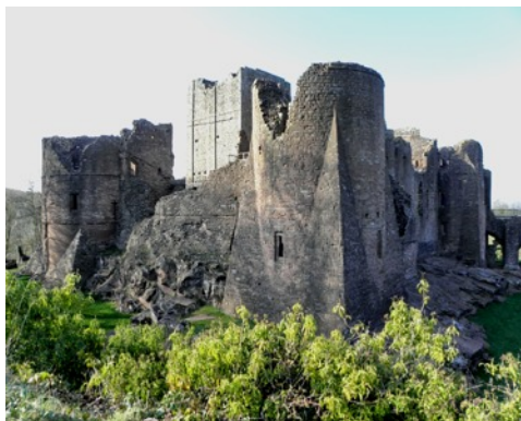
Fig. 24. Goodrich Castle from the south. The great tower, c. 1148, centre, within the courtyard of the later quadrangular castle and behind an 'en bec' enceinte.
