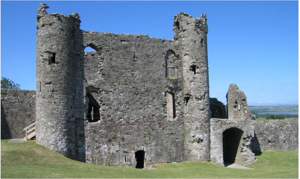
Fig 45. Llansteffan. The 1260s gatehouse from the south, from inside the lower ward. The main entrance was blocked in the Tudor period. The present entry point via the wooden stairs may not have been the original. Unlike Tonbridge and Caerphilly the stair-turrets here are solid from the basement to the first floor.
