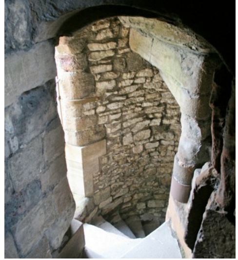
Fig. 87. Dudley Castle. A view of the anticlockwise newel rising from the basement into a small lobby. To the left is the start of the clockwise spiral up to the wall walk.
