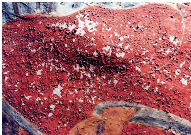
FIGURE 2 Blistering and disruption of wall painting in cave 35, Mogao Grottoes, Dunhuang.
