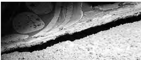
FIGURE 4 Plaster detachment of wall painting in cave 6, Yulin Grottoes, Dunhuang.
