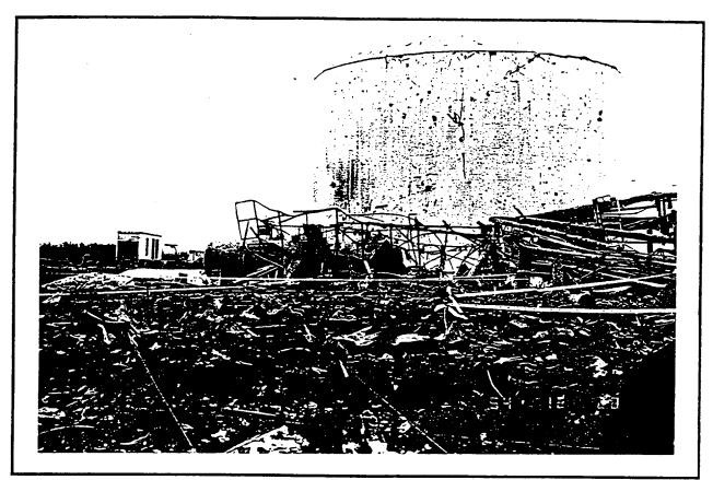
Photo 8 - 12 Water Tank Damage (Ammonia Tank Background)
