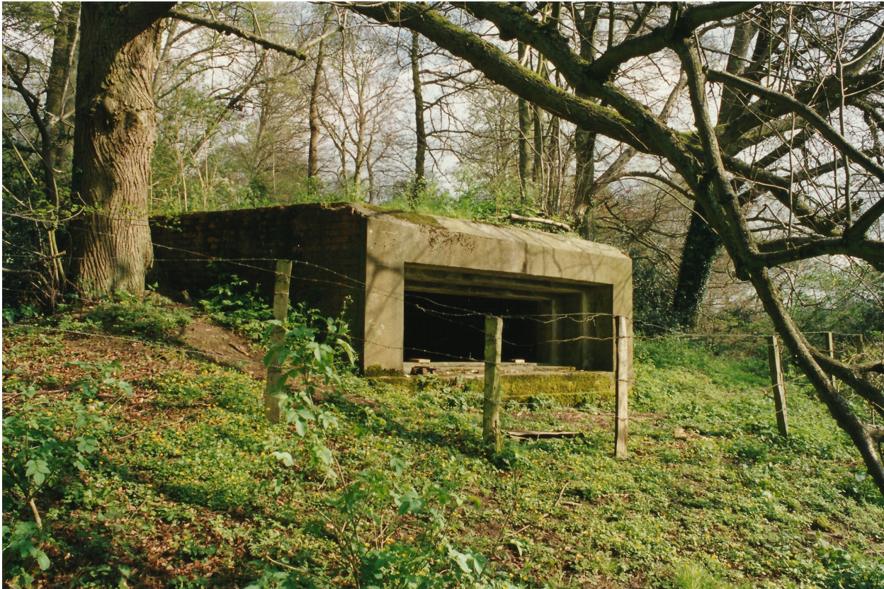
Anti-tank gun emplacement, Moor Park, Farnham.
