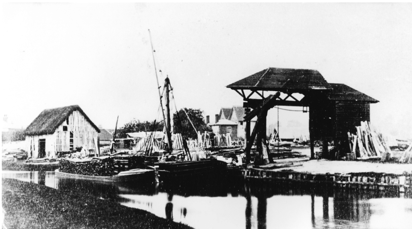
Stonebridge wharf, Shalford, on the Godalming Navigation, 1915, showing the gunpowder store (left) and treadwheel crane (right).
