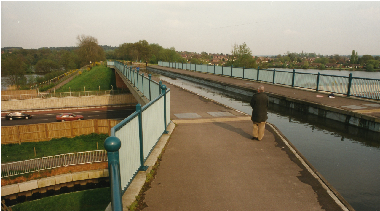
The aqueduct carrying the Basingstoke Canal over the A331 Blackwater Valley road opened in the 1990s.
