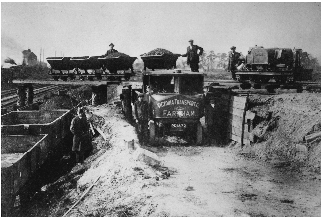
Gravel extraction at Weydon Lane, Farnham, early twentieth century.
