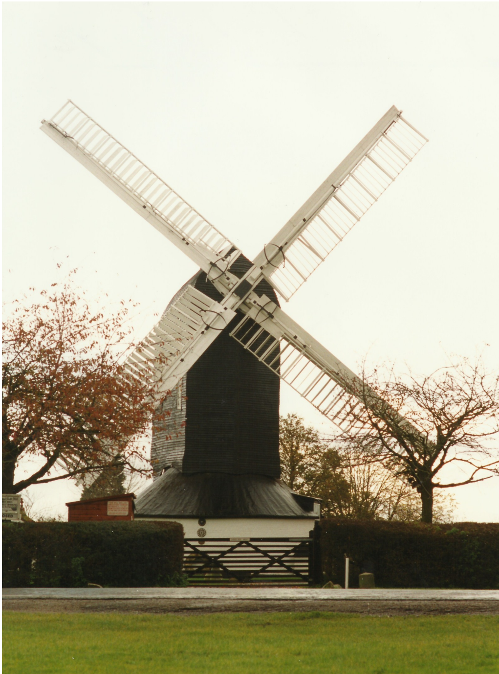
Outwood post mill.
