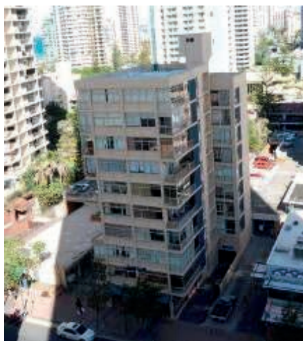
Kinkabool High Rise Apartments (© GCCC 2010)
