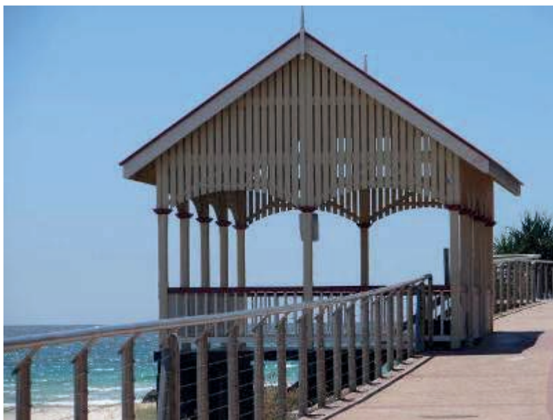
Kirra Shelter Shed (© GCCC 2009)
