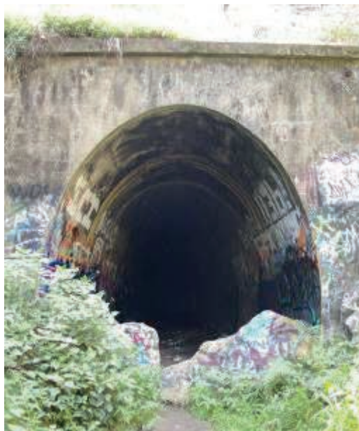
Western entrance, Ernest Junction Railway Tunnel (© GCCC 2010)
