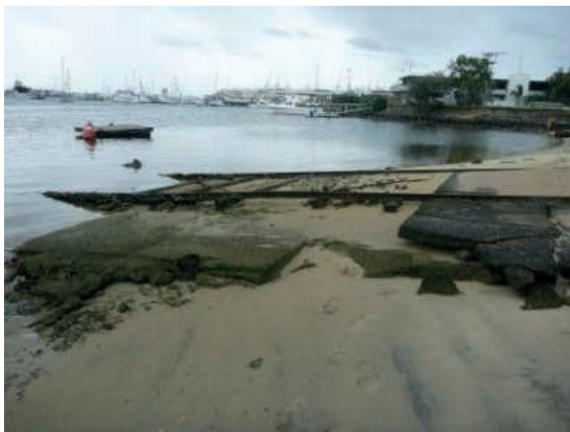
Humphreys Slipway, Main Beach (© GCCC 2010)
