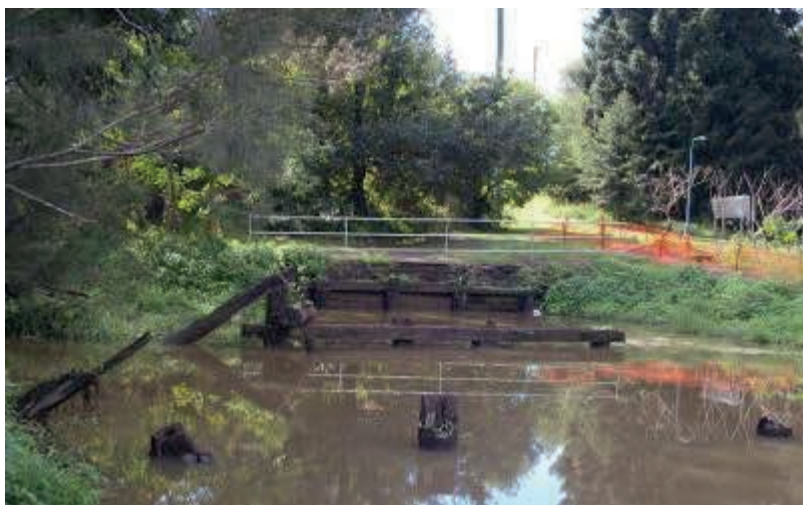
Dip Crossing Bridge remnants, Mudgeeraba Creek (© GCCC 2011)
