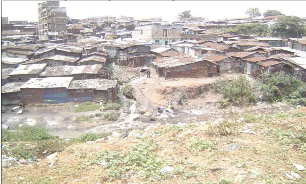
Photo 3.2 Housing and drainage in Kosovo Village, Mathare Slum
