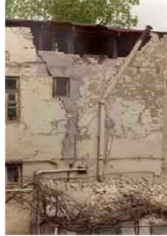
Fig. 8. Failed brick wall
