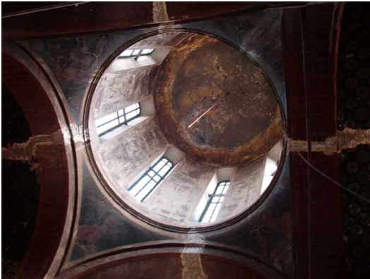
Fig . 5. Repaired symmetrical cracks, 300 Aragveli church. Fig. 6. Shifted and overturned monuments in grave yards
