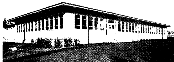
An attractively designed temporary wood, frame and stucco building has been added to the parking-lot area East of the University Armoury to house the University's new College and Faculty of Education until permanent quarters can be constructed later.
