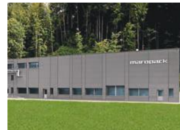
Rommelag state-of-the-art contract BFS production facility in Zell, Switzerland supports Bio-safety Level 2 processes.
