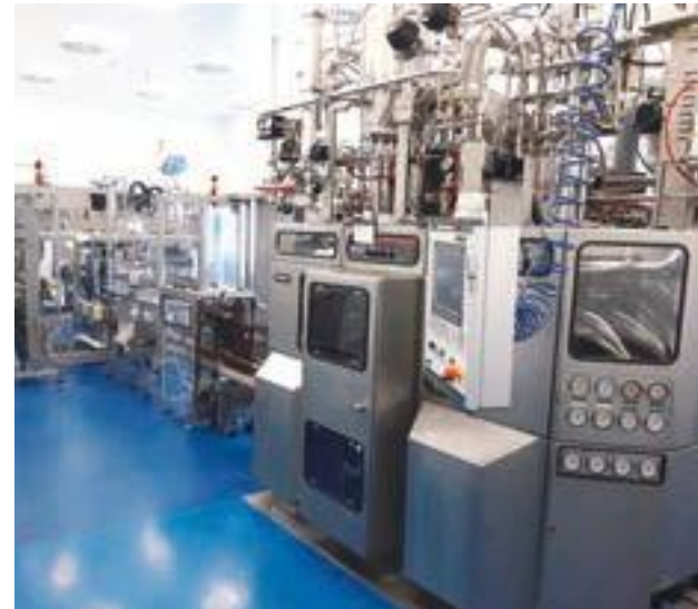
BFS machines are compact. This allows 6-8 machines in a 100,000 sq. foot facility to produce a billion sterile BFS doses a year.
