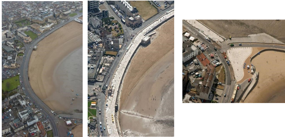
Aerial views 2002 (left) and 2009 (middle) showing paving and walling work almost complete and right Marine Lake Plaza in 2009 with new feature paving (compare with bottom right of 2002 photo)
