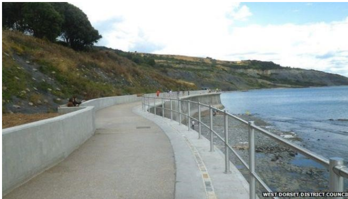
Lyme Regis Phase IV East Cliff scheme completed in 2015
