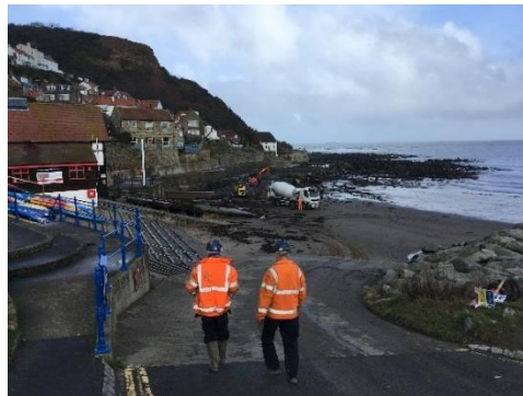
Runswick: Construction works to sea wall
