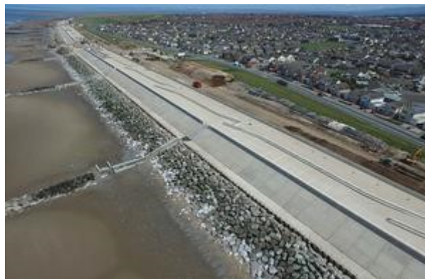
The Rossall coastal defence scheme, opened on 1 June 2018
