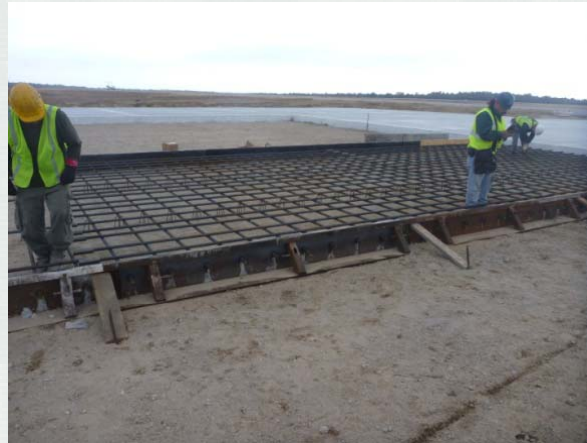
Rebar placement of interior lane
