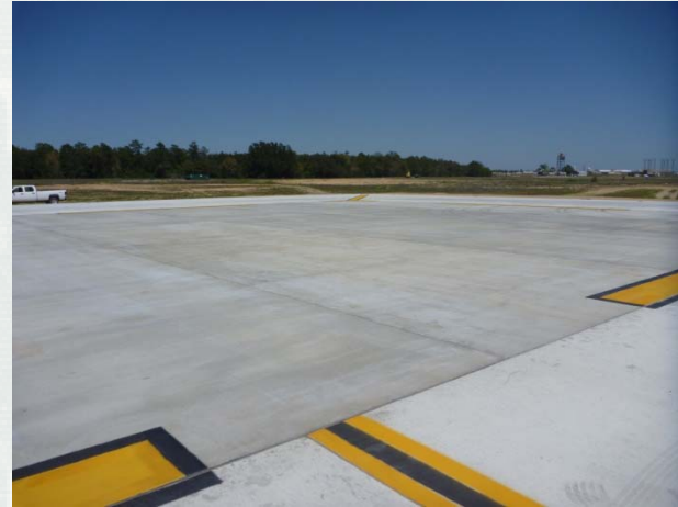
Sodium silicate application
