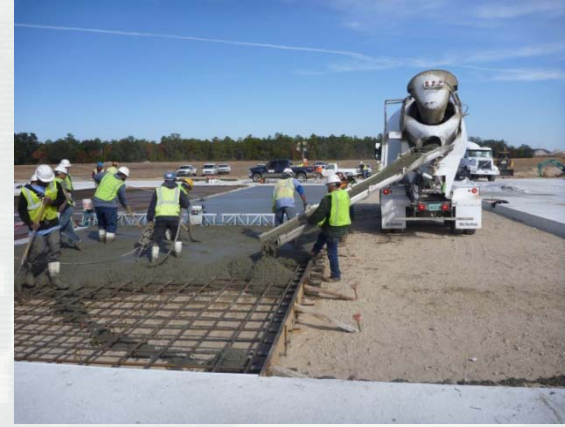
Concrete placement – emergency tailgating interior lane
