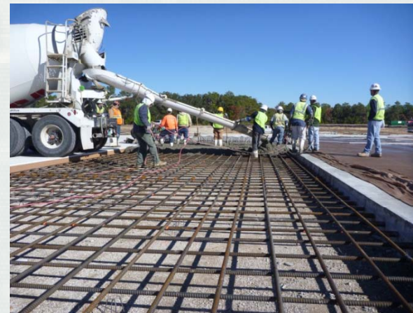
Concrete placement – tailgated
