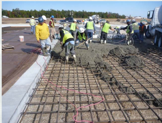
Concrete placement – emergency tailgating interior lane
