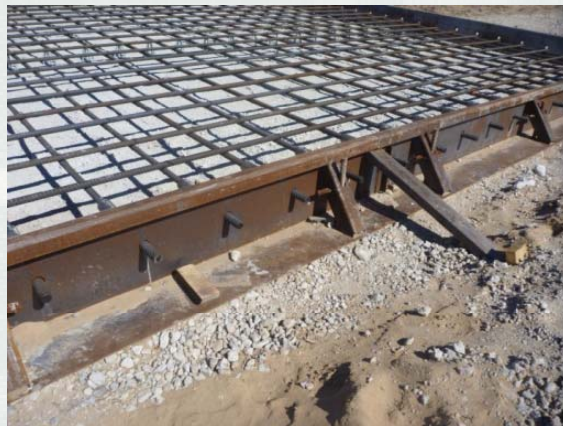
Rebar placement of exterior lanes
