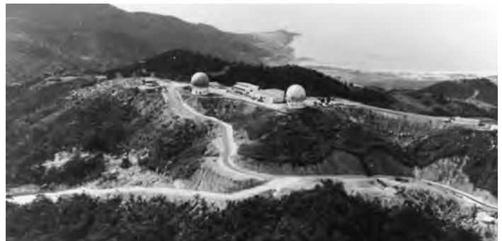
Operations site of the 6924 SS, Da Nang, South Vietnam in 1966.
