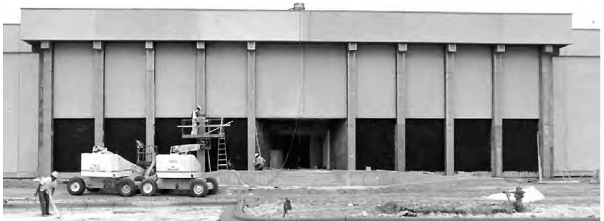
Construction on building 2007, January 1986.
