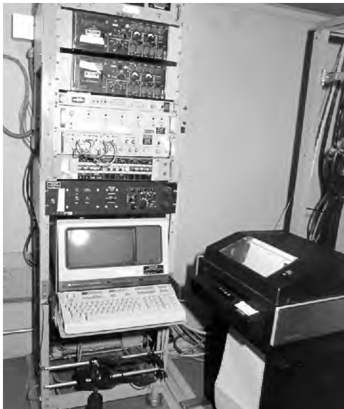
Interior of Comfy Shield "I-Hut" of the 6948th ESS.
