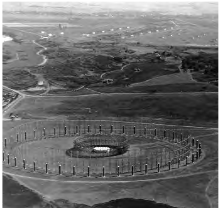
AN FLR-9 and Operations building at the 6922 SS, Clark AB, Philippines.
