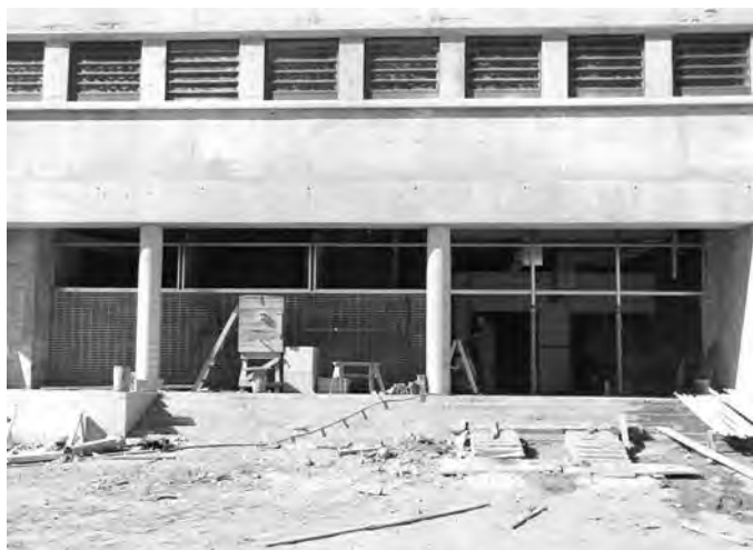
Construction of the front of Bldg. 2000--later known as Ardisana Hall--winter 1952.
