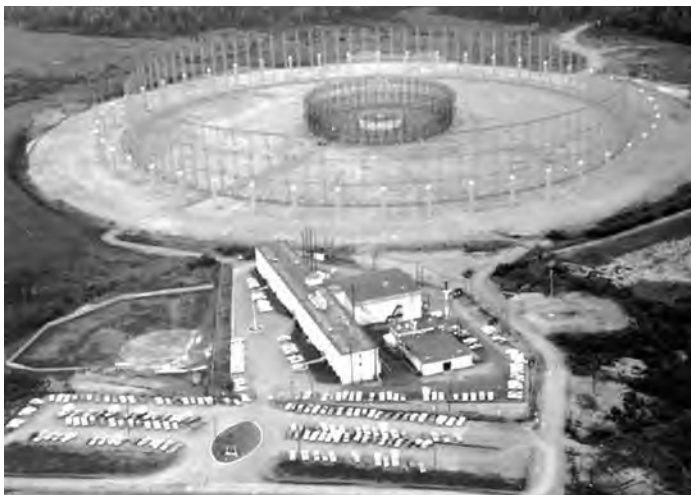
By the mid-1960s AN FLR-9 "Elephant Cages" became the mainstays of several USAFSS units, including this one at the then 6981st SS, Elmendorf AFB, AK.
