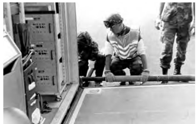
Members of ESC's 6948th ESS assemble the floor brace of a Comfy Shield Hut at Border Star-85, March 1985.
